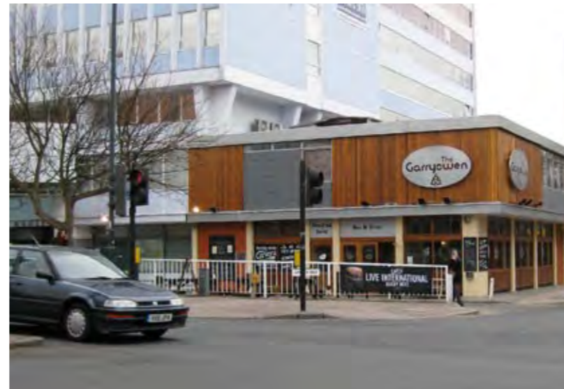
Ground floor restaurant/bar uses at Regal House, with office accommodation above
