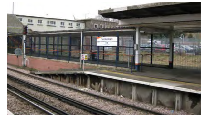
The existing platform arrangement
