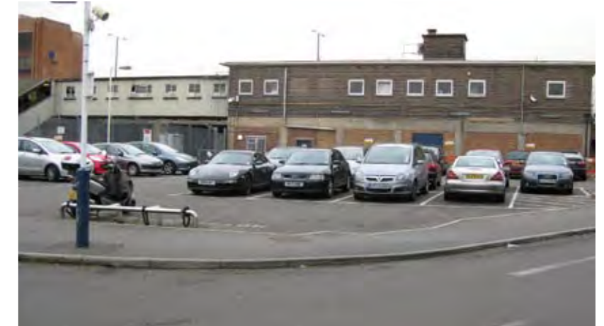
Existing poor quality buildings on the site
