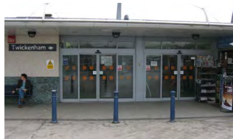
The existing station entrance on London Road
