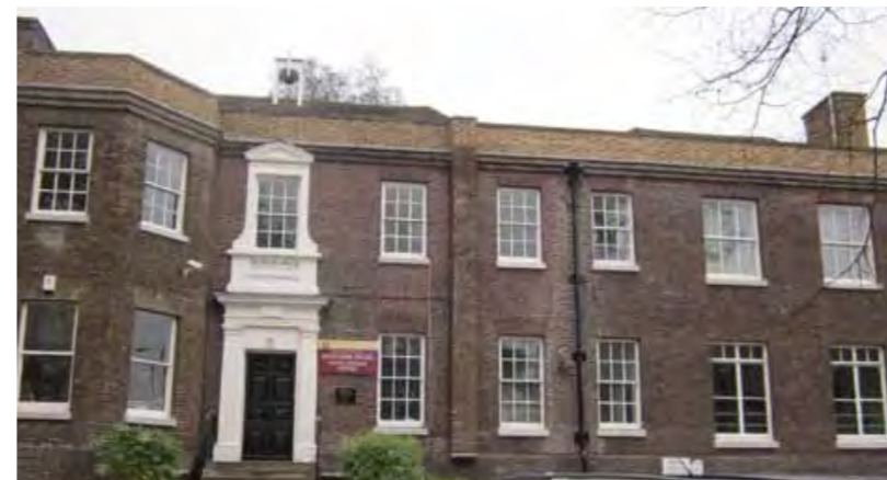
Figure 3.11 Top: Richmond Hill terrace Bottom: Heatham House
