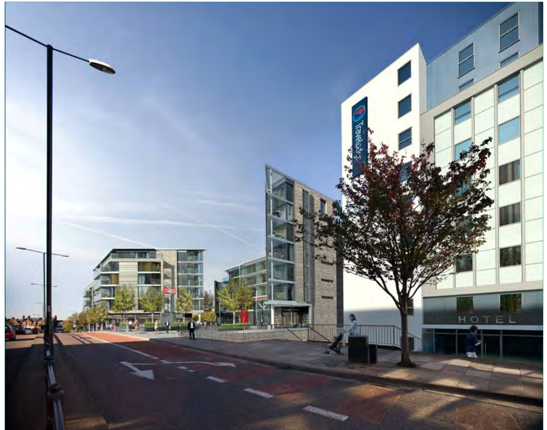
Figure 4.2 The station viewed from London Road
