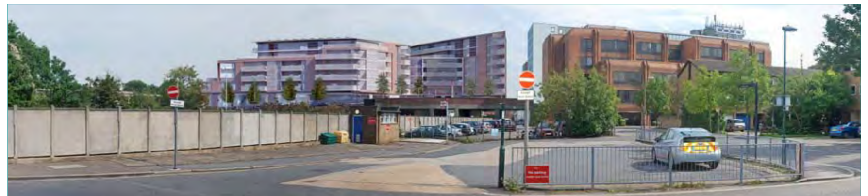
Figure 4.13 Photo montage of the site looking east from The Albany public house, Queens Road
