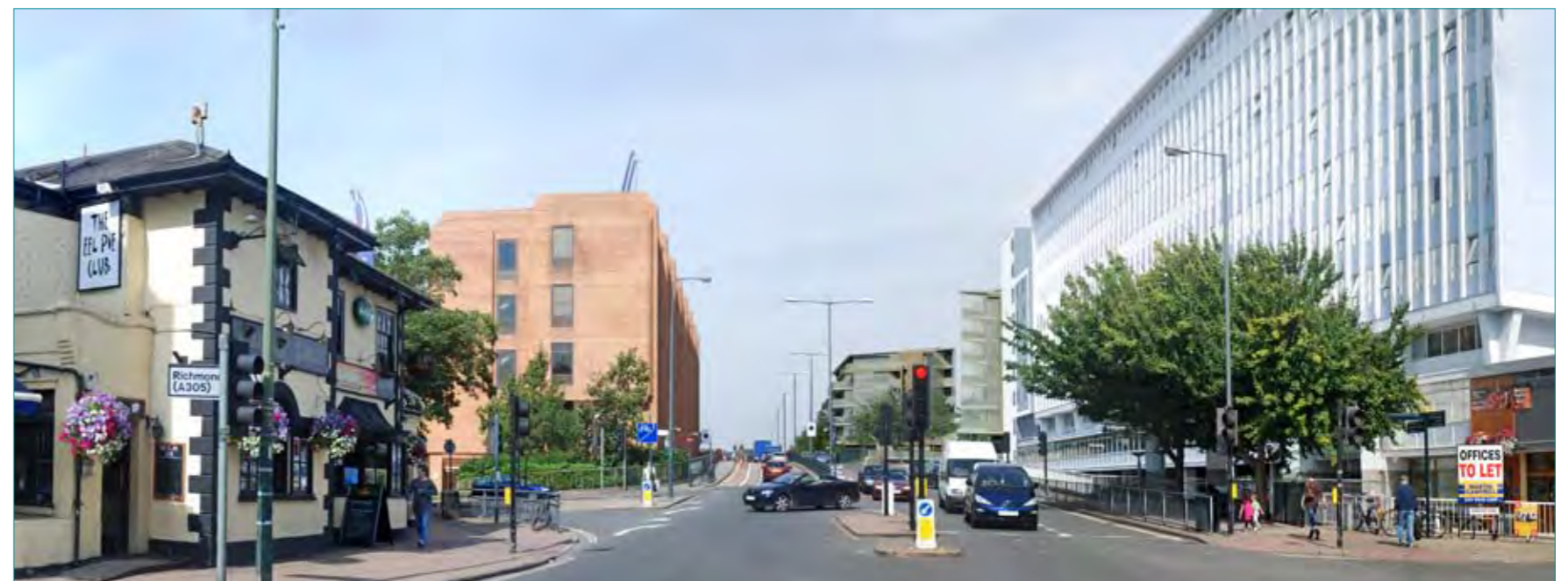
Figure 4.14 Photo montage of the site looking north from pedestrian crossing at junction of Arragon Road and London Road.
