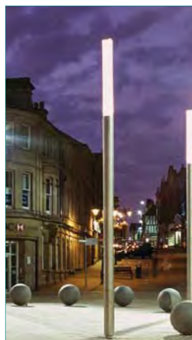
Column lights providing security lighting at podium level
