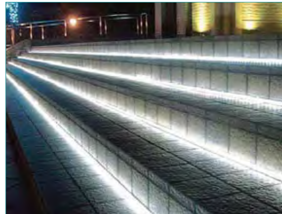
recessed step lighting
