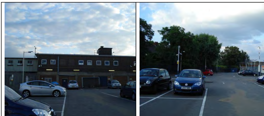
Plates 13-1 & 13-2 View of station building and associated car parking facility.
