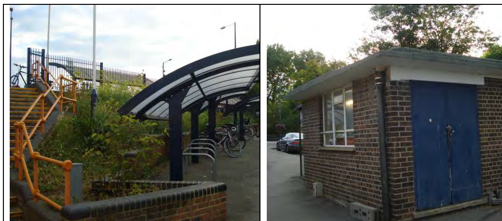
Plate 13-3 and Plate 13-4 View of bike shed in the north west of the site and View of small building adjacent to bike shed.
