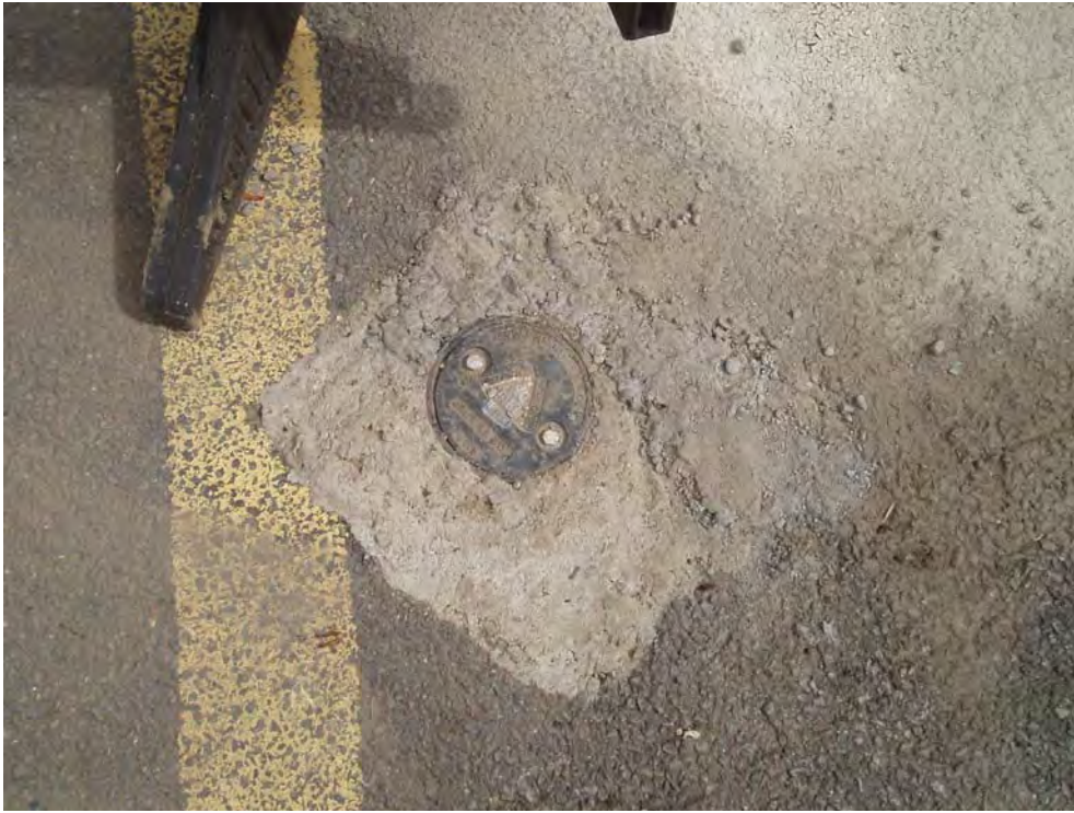
Plate 3: Cover of finished cable percussion borehole BHF.
