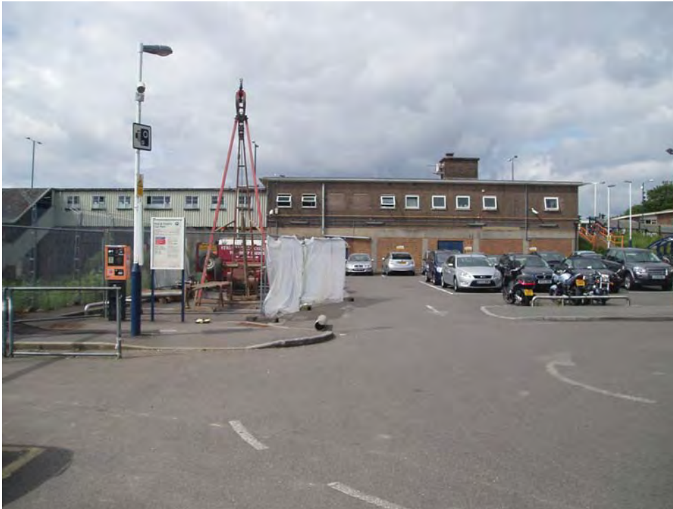
Plate 1: Cable percussion drilling of Borehole BHD.
