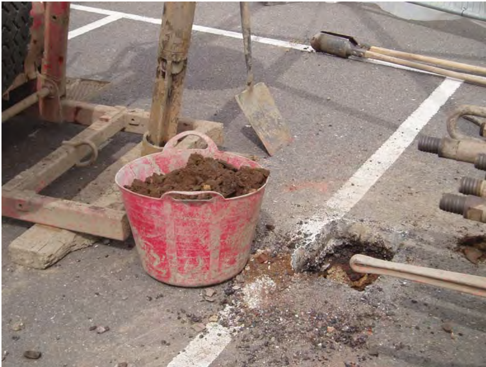
Plate 6: Location of open cable percussion borehole BHD with drilling spoil.
