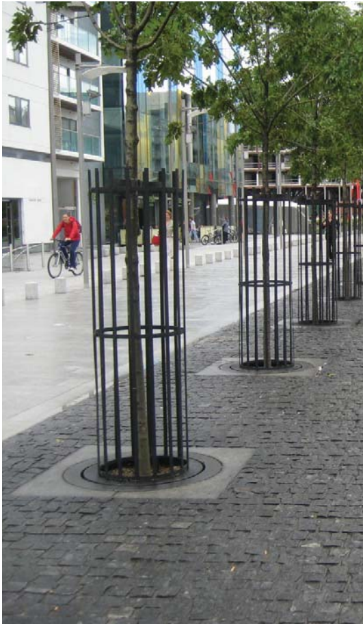
Metal tree guards to Riverside Square
