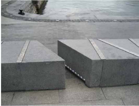
Downlighting to seats
