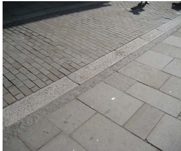
Small size units indicate vehicular routes, in contrast with larger units to pedestrian areas, separated by edgings or low kerbs
