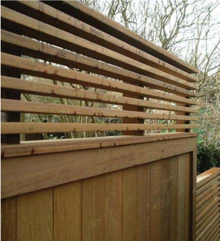
Robust horizontal rail timber screen to edge of riverside square, ht 1.2m
