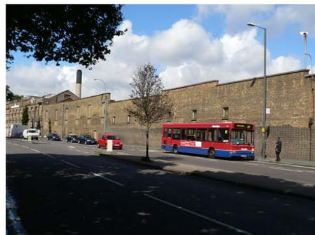
Fig 3 : Boundary wall to Stag Brewery Site
