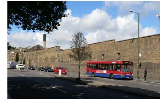
Fig 8: Stag Brewery wall & public highway (to North of site)
