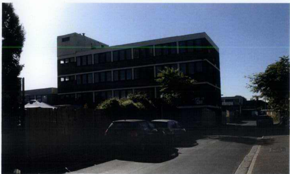
10. IMX House prior to demolition
