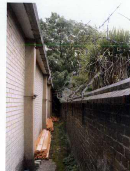
12. Existing southern boundary wall and dairy building
