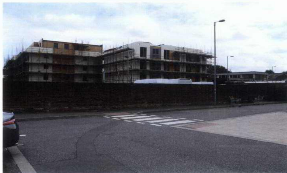
4. Approved Garden Road development under construction from Sainsbury's car park
