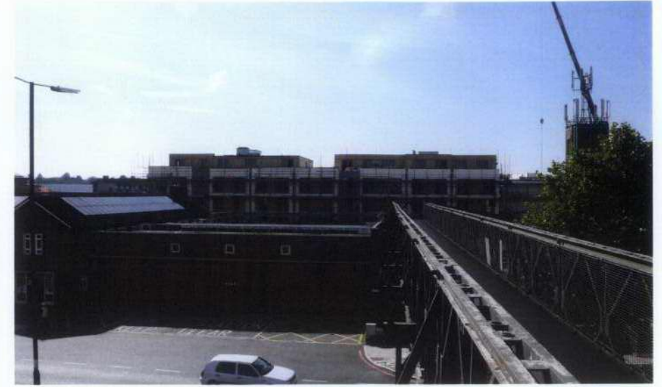
3. Approved Garden Road development under construction from footbridge over A316
