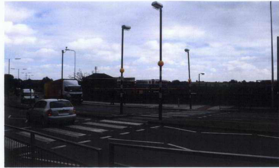
2. View from Manor Circus with approved Garden Road development under construction
