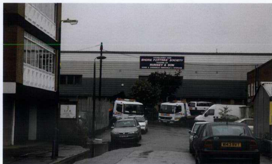
11. Rumsey and Son building on Market Road
