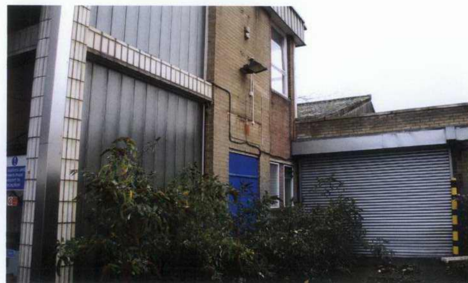
4. Existing dairy building
