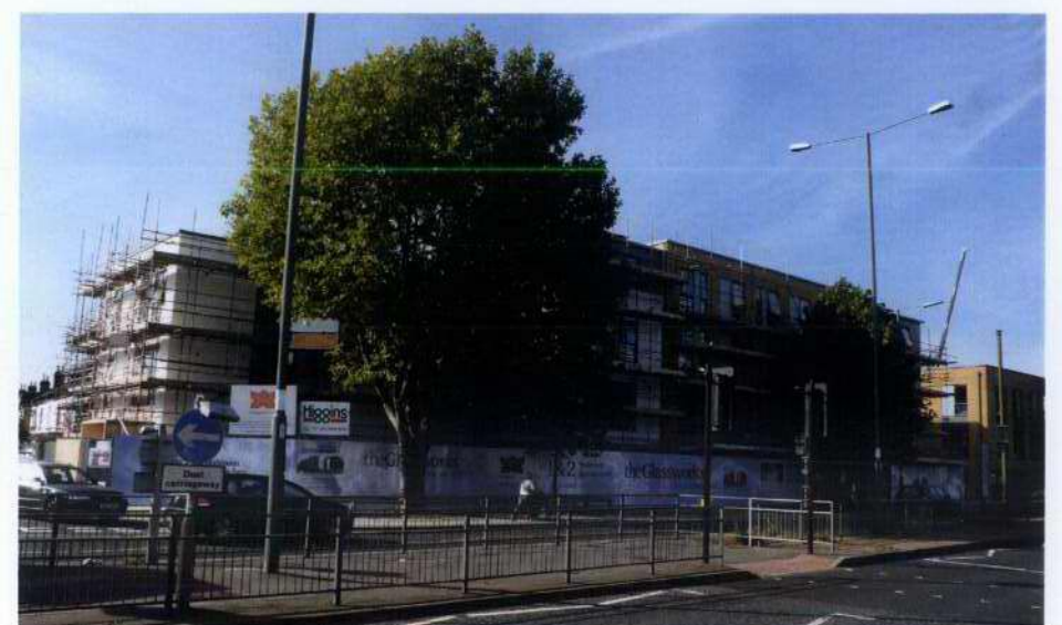
12. The Glasshouse development currently under construction
