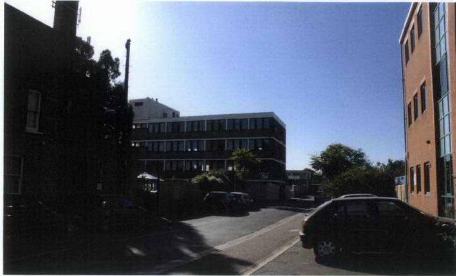
1. Orchard Road looking south to site past IMX House prior to demolition
