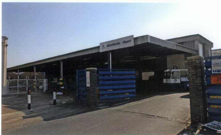
3. Existing dairy building from north west corner of the site
