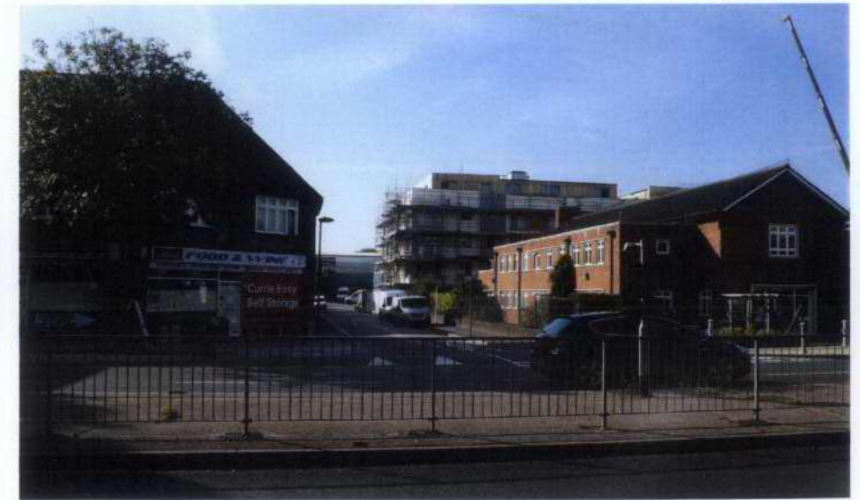
6. View down Market Road from the A316
