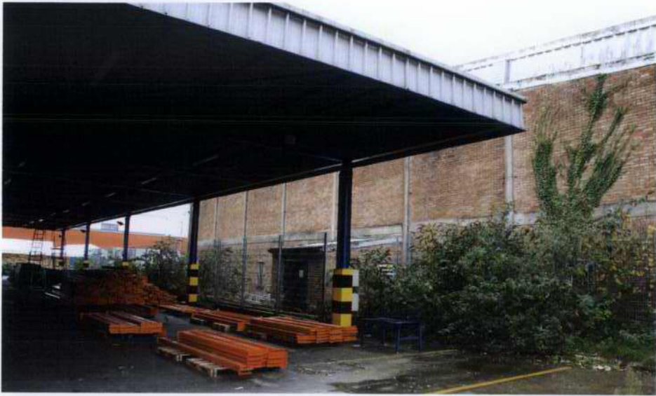
7. Service yard with IMX House prior to demolition in the background
