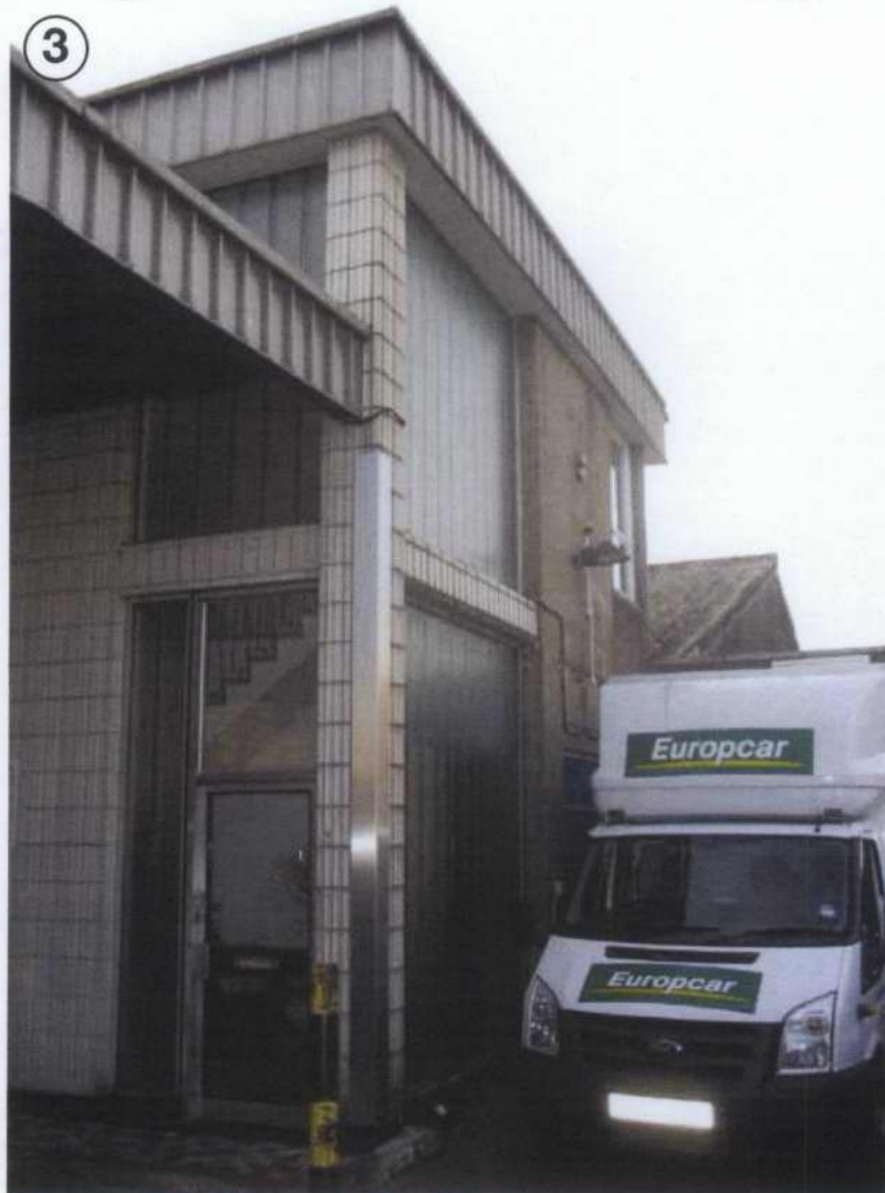
Photograph 3 - View of South-West corner of building looking South
