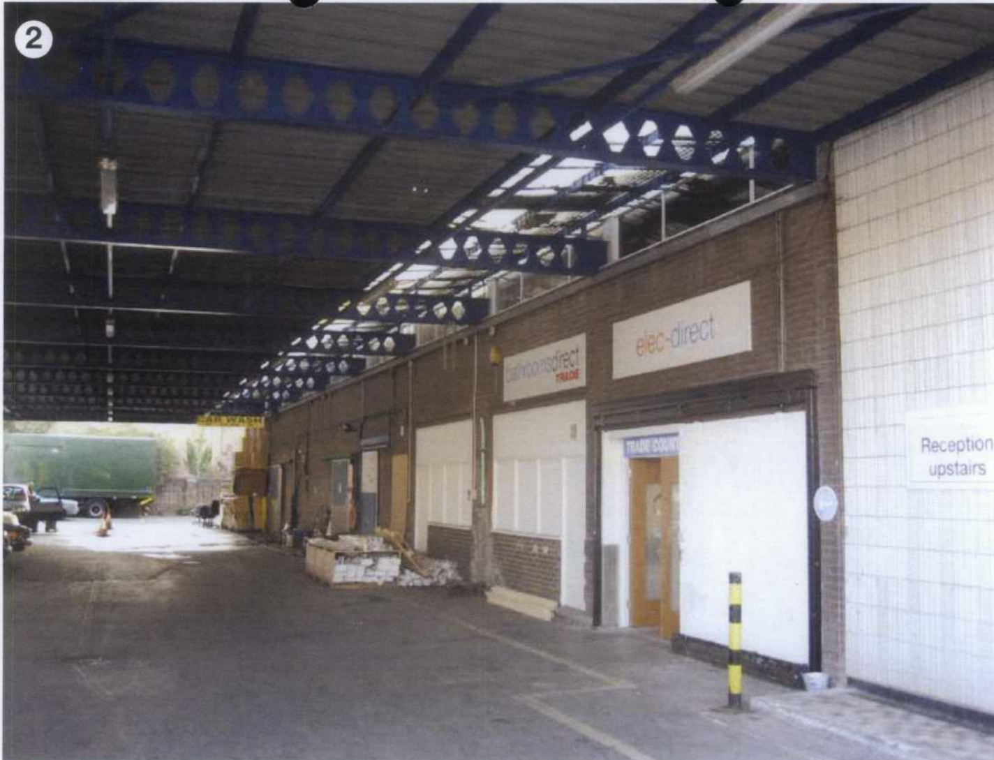
Photograph 2 - View of ground floor elevation looking West
