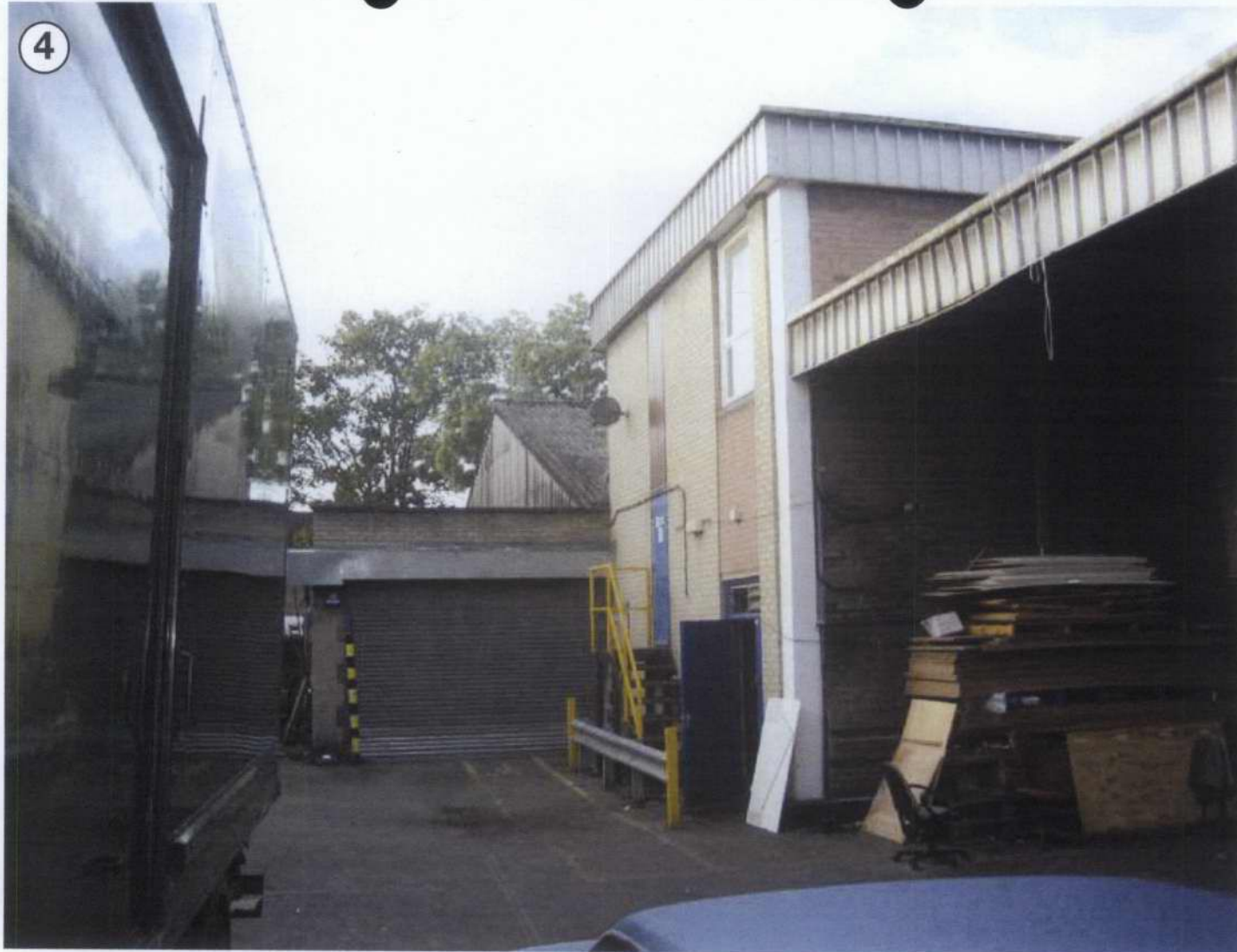
Photograph 4 - View of South-East corner of building looking South
