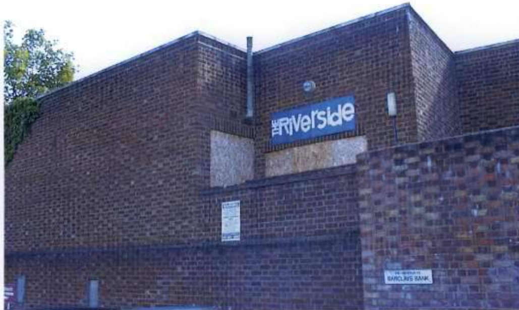
Plate 19 - Restaurant - Cement flue to northeast corner
