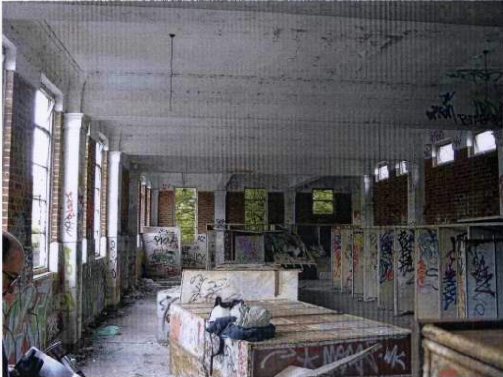
Plate 1 - Interior view of the main building
