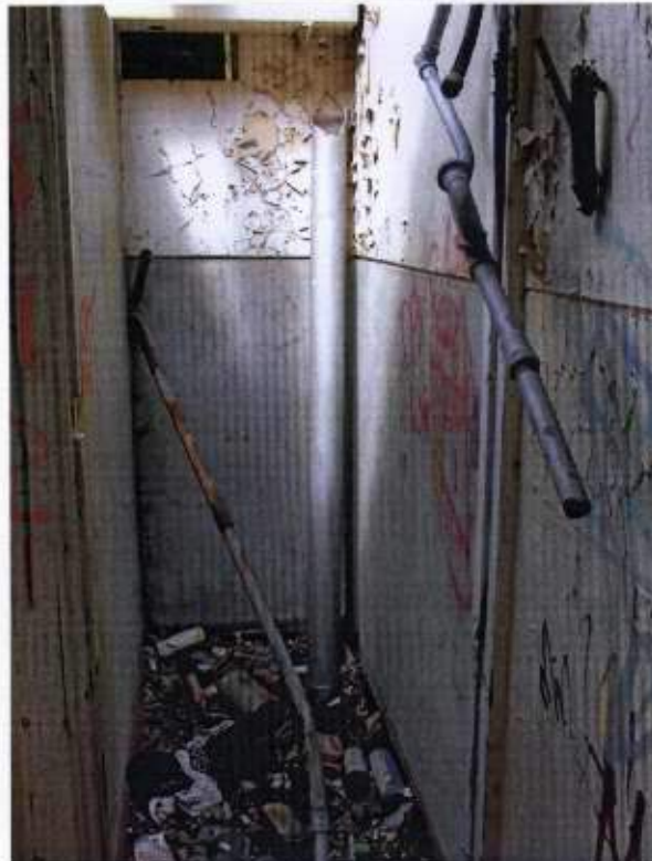
Plate 5 - Changing Block - redundant cement flue/pipe in ladies WC (East Toilets)
