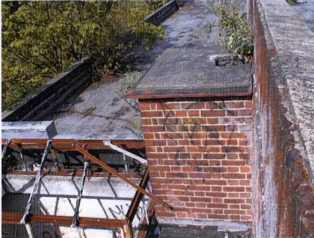
Plate 15 - Changing Block - stack to northwest elevation
