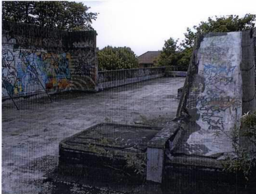
Plate 11 - Changing Block - bituminous screeds and felt to roof
