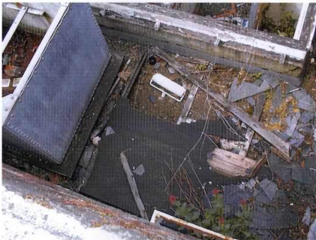
Plate 12 - Bituminous felt to roof of ladies WC (East Toilets)
