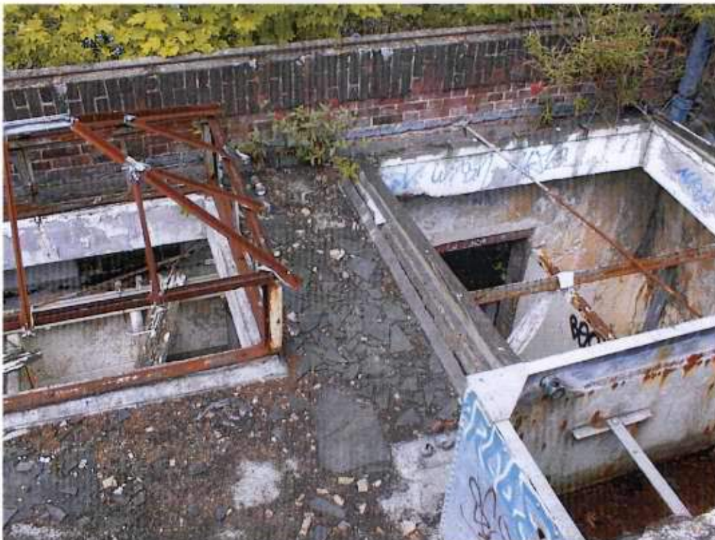
Plate 16 - Changing Block - skylight above ladies WC (East Toilets)
