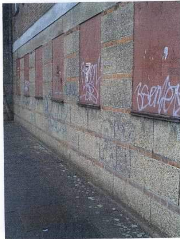
Pool building wall and window, which will be demolished to make way for proposed garden.
