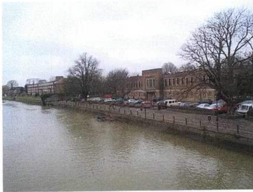
View of Twickenham Baths site from Eel Pie bridge.
