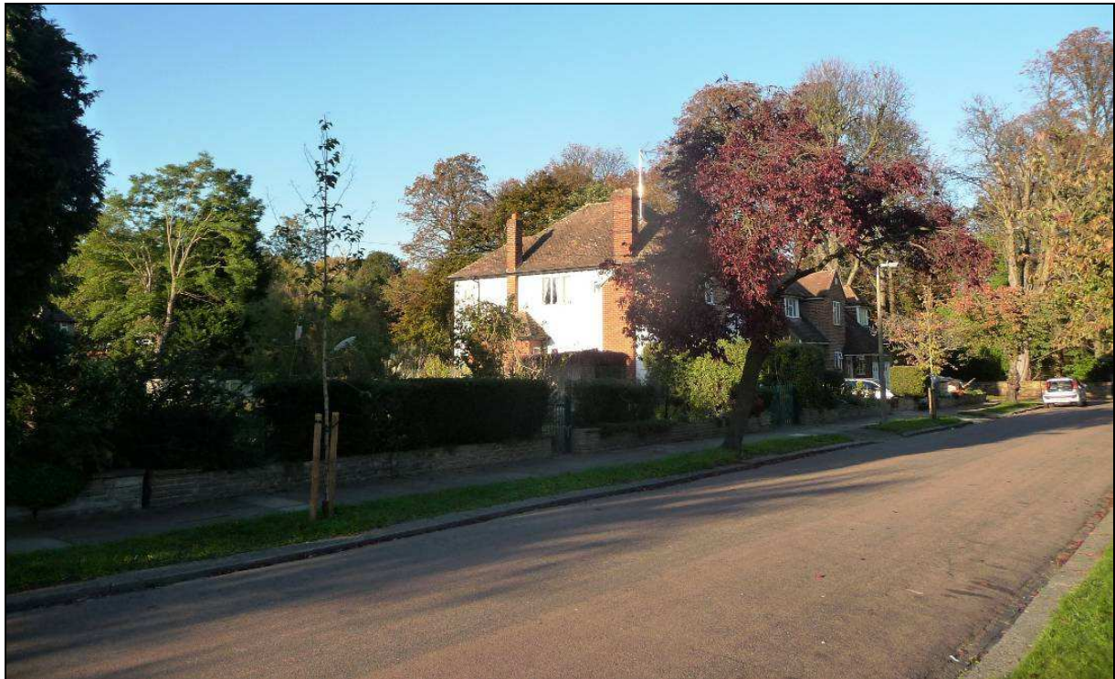
Photo 2: View north across Melbourne Road towards site
