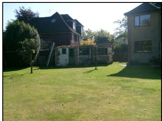
Garden/garage in rear garden
