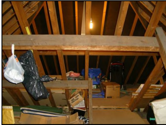
Internal loft space
