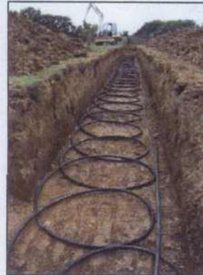
External Collection Trench
