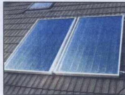
Flat Plate Collectors
