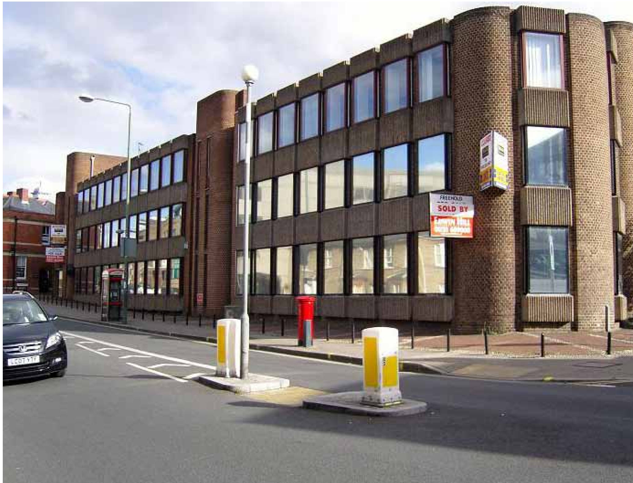
9-19 Paradise Road - Existing Office Building
