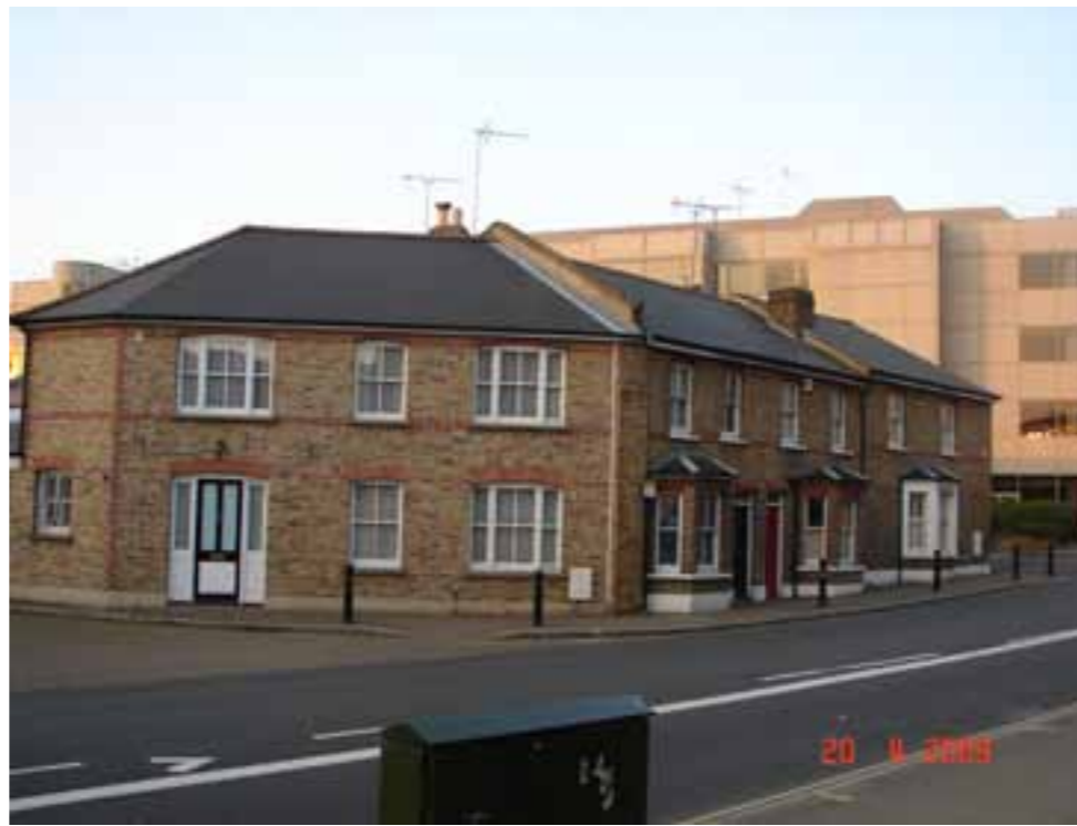
New residential development opposite
