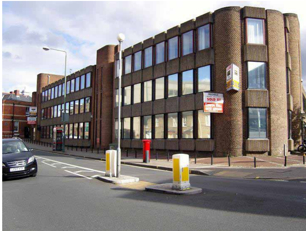
View looking East along Paradise Road
