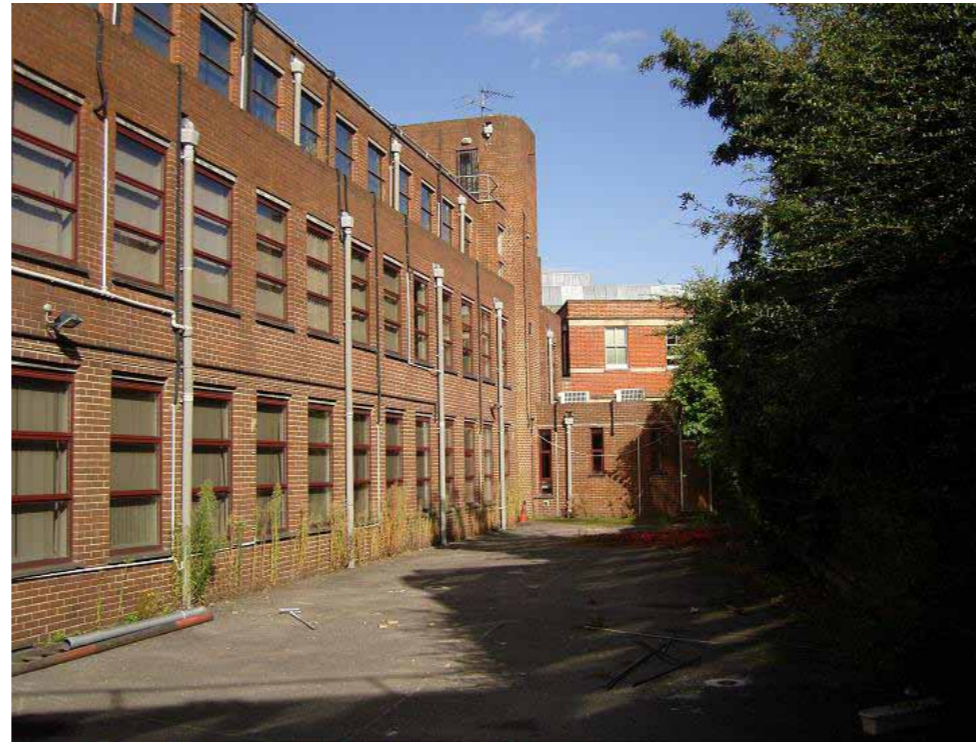
View of rear yard and back elevation
