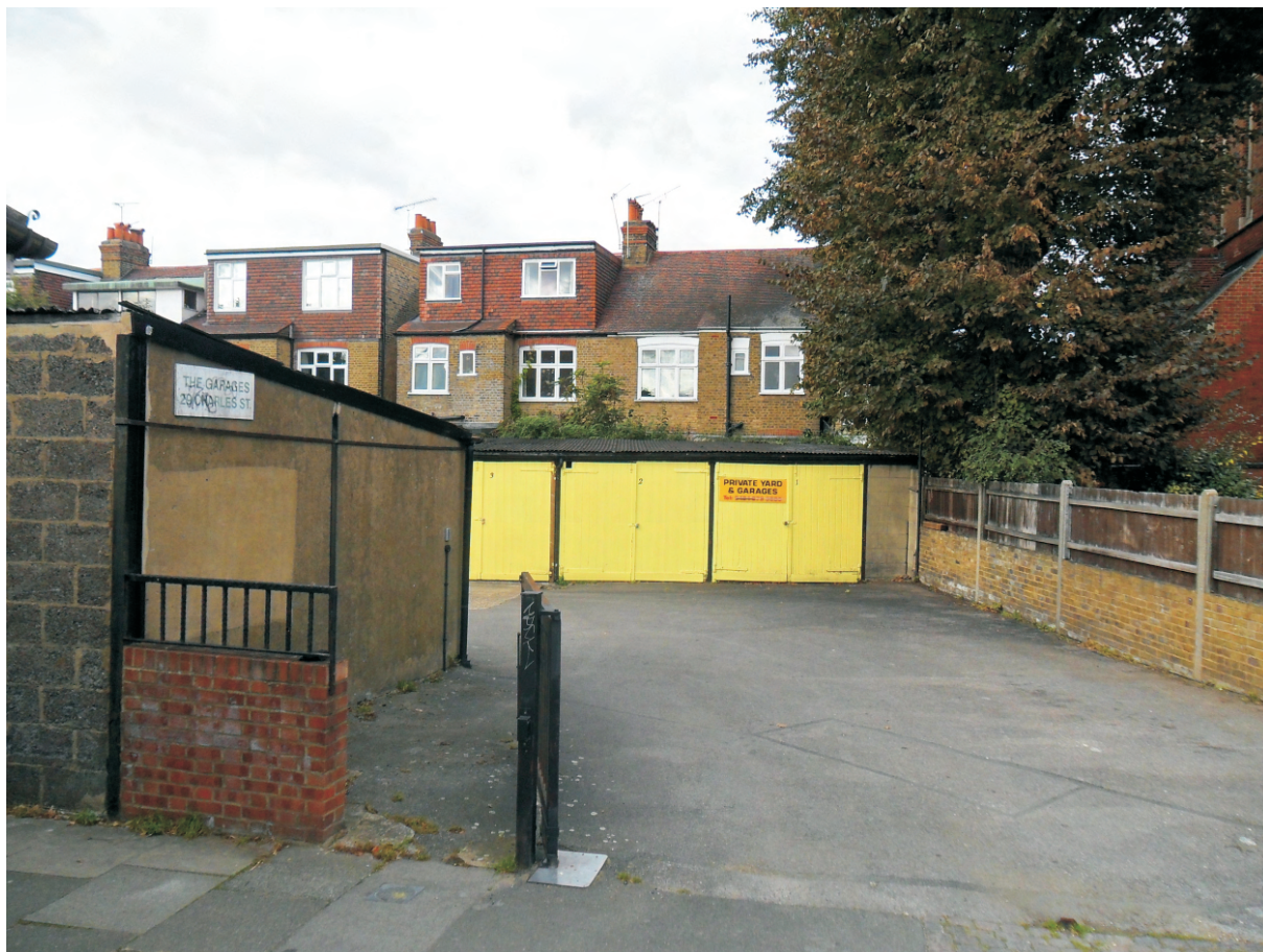
Plate 1: The Garages 29 Charles Street entrance
