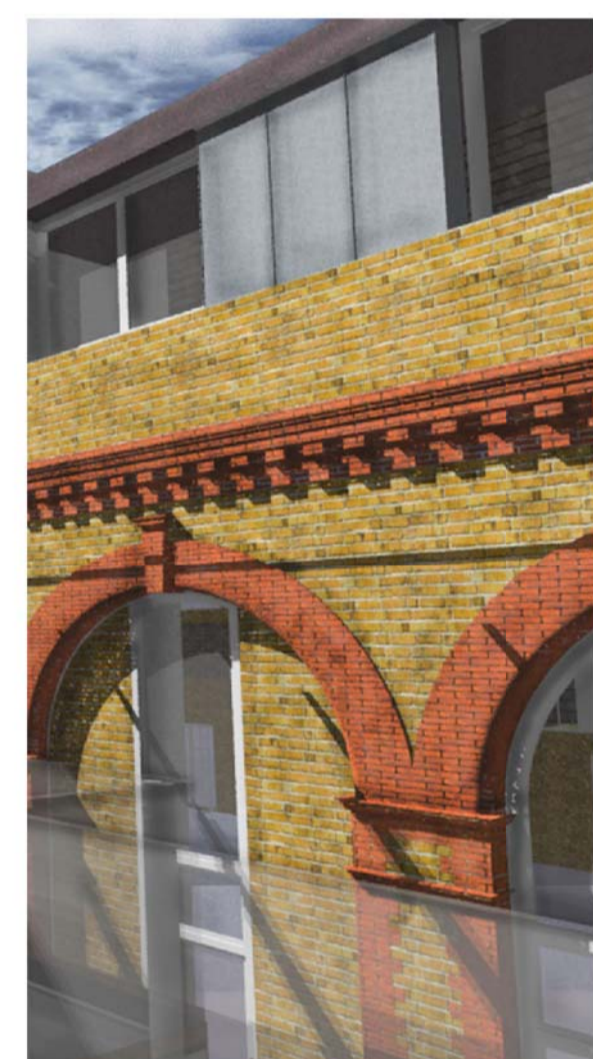
Brick dentil courses and decorative arches to be retained in courtyard and cleaned.
