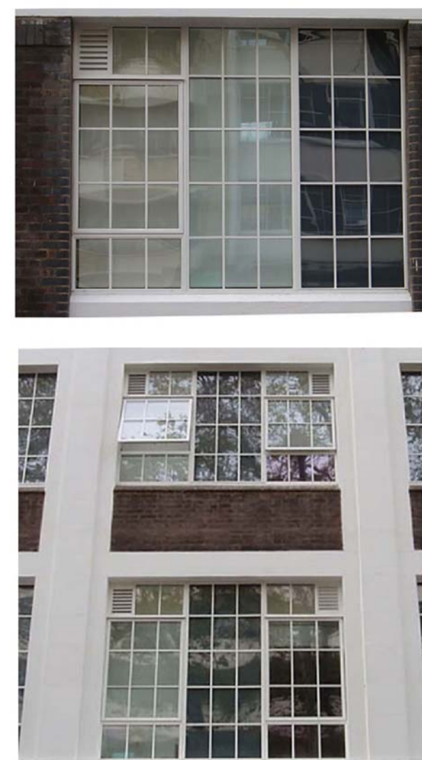
Example of replacement metal window
