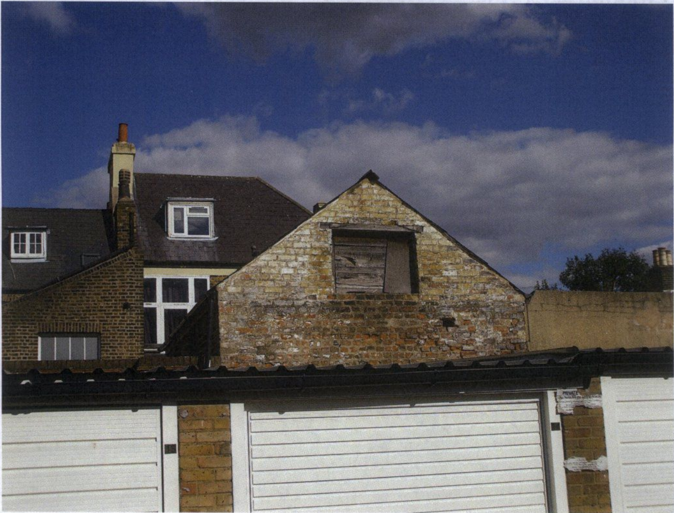
Fig 5. Rear of stable building visible
