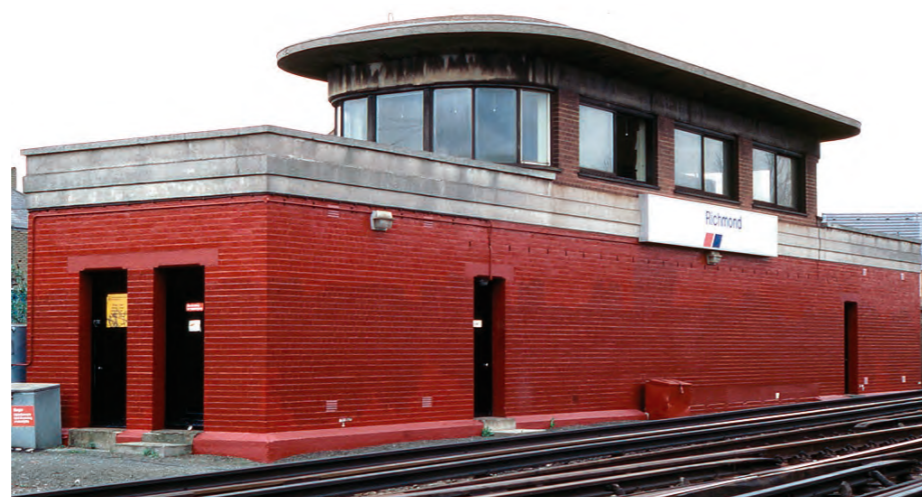
Richmond signal box
