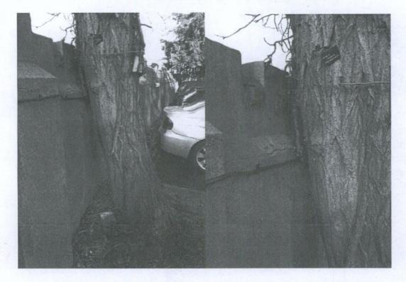
As the area of conflict is at the top of the wall and it direct contact with the stem, we are not able to offer an engineering solution that does not affect the appearance of the wall.
