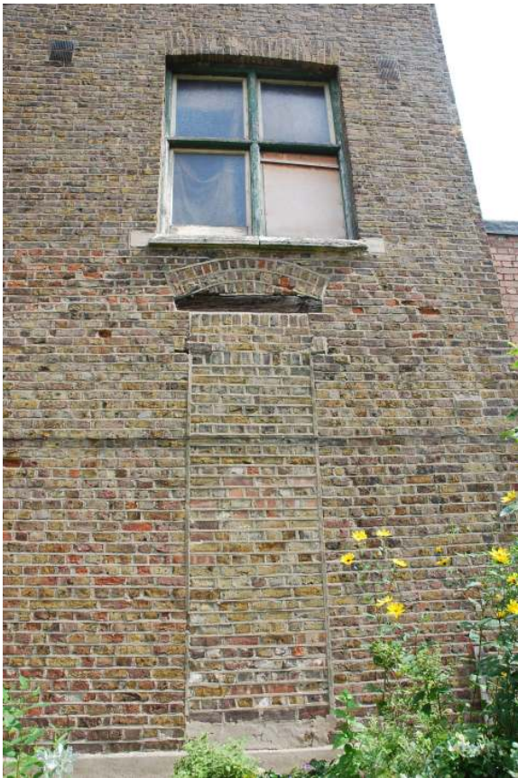
Fig.22: Blocked doorway in SW corner of former Auditorium/ Town Hall
