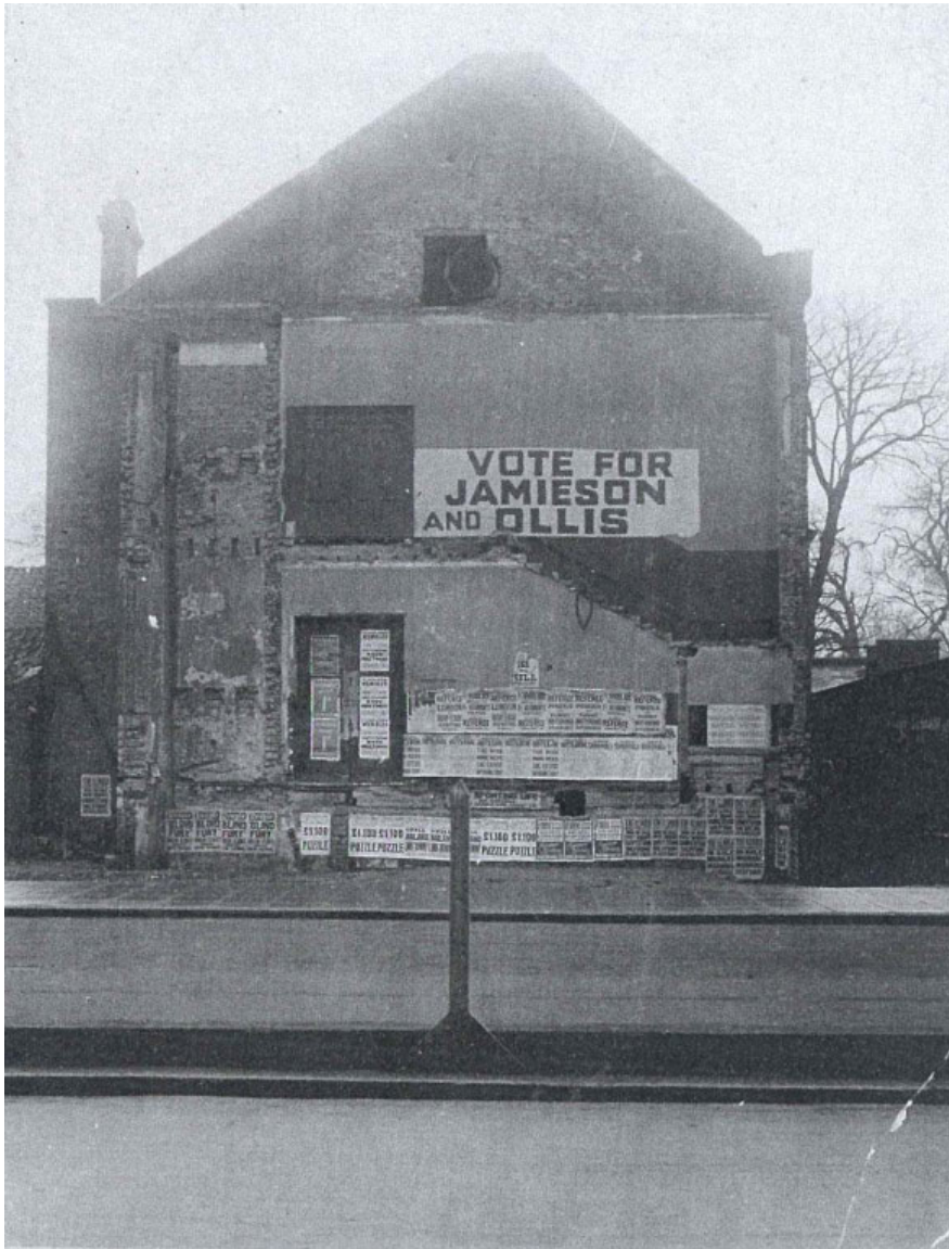
Fig.9: King Street after road widening showing the exposed north end of the Auditorium, now known as Queens Hall. Pre-construction of the new parade of shops
