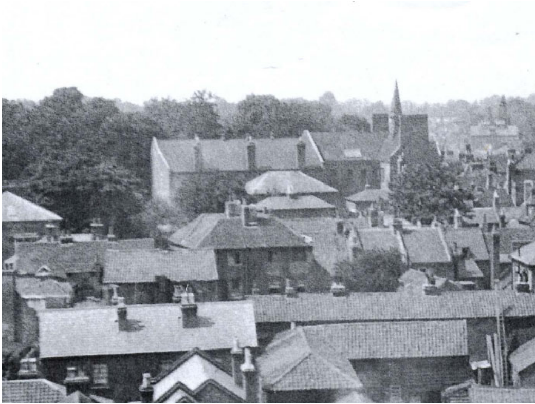
Fig. 15: Photograph showing the Town Hall as was c.1920
