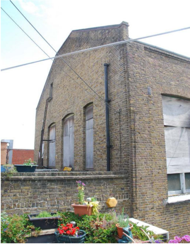
Fig.20: NW corner of former Auditorium building, facing SE, showing roof terrace between King Street frontages and Queens Hall
