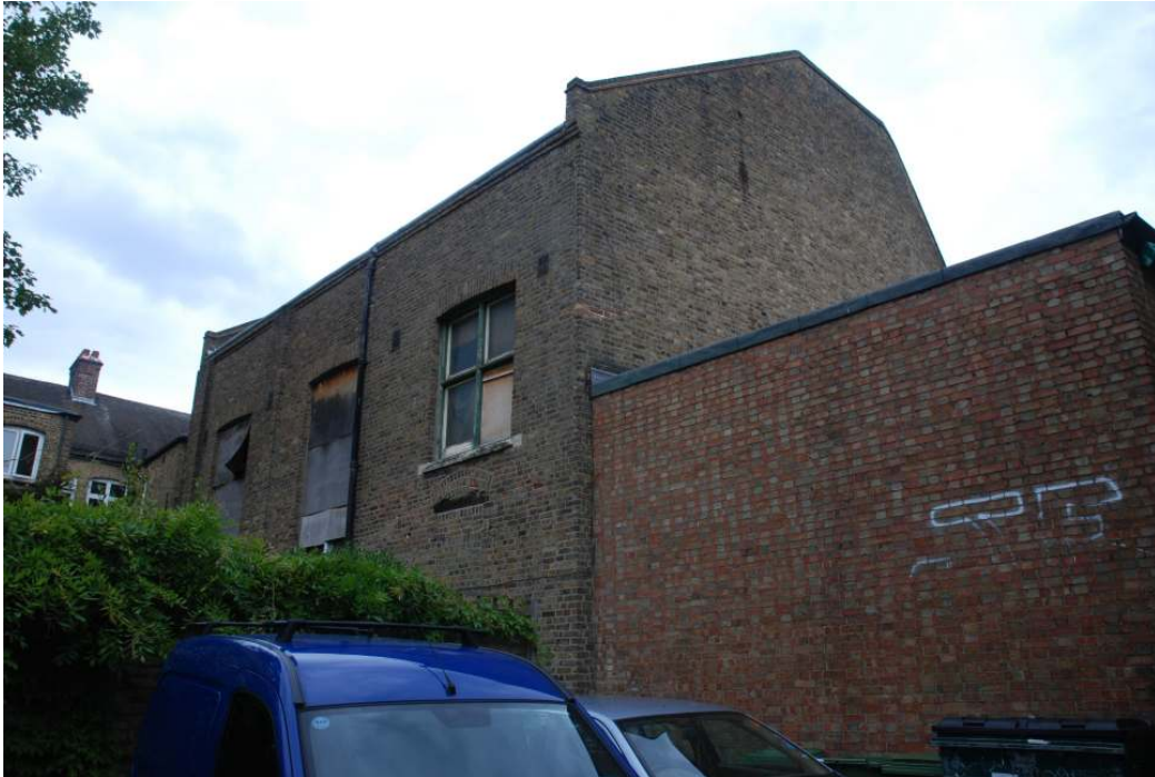
Fig..21: West side of former Auditorium/Town Hall, facing NE
