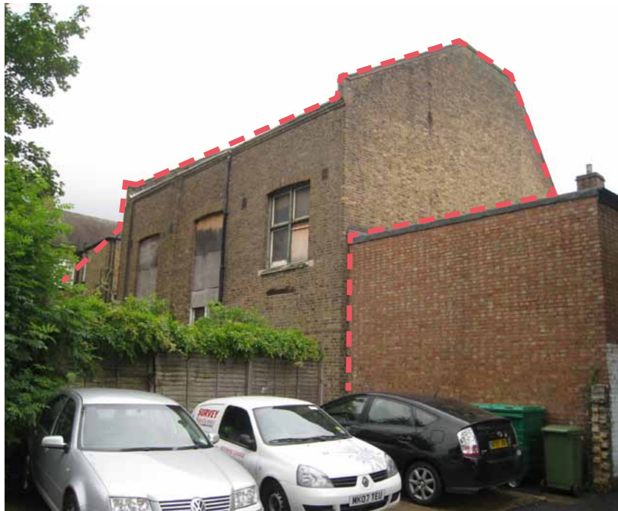
Queens Hall view of existing west elevation
