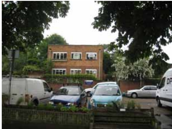
View 2 taken from river walk looking north, Primary view along River Thames unaffected. Queens Hall not visible over existing building in foreground. No change during winter months.
