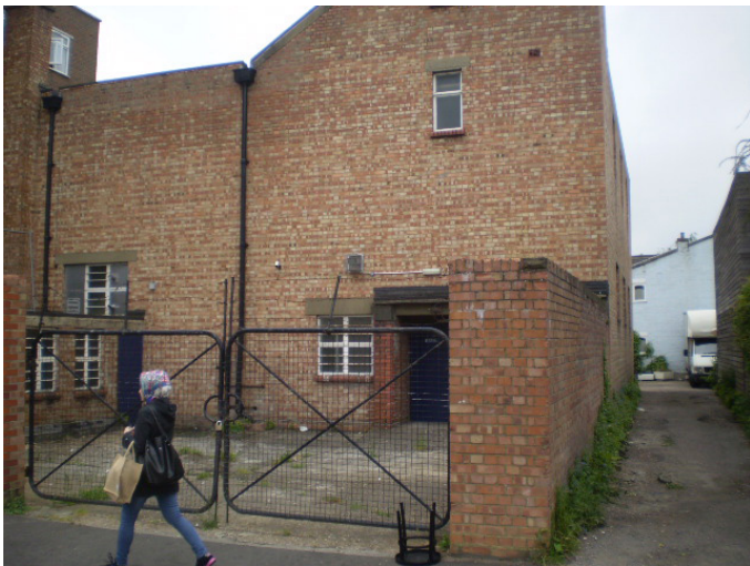
Existing rear service yard accessed off Elfin Grove
