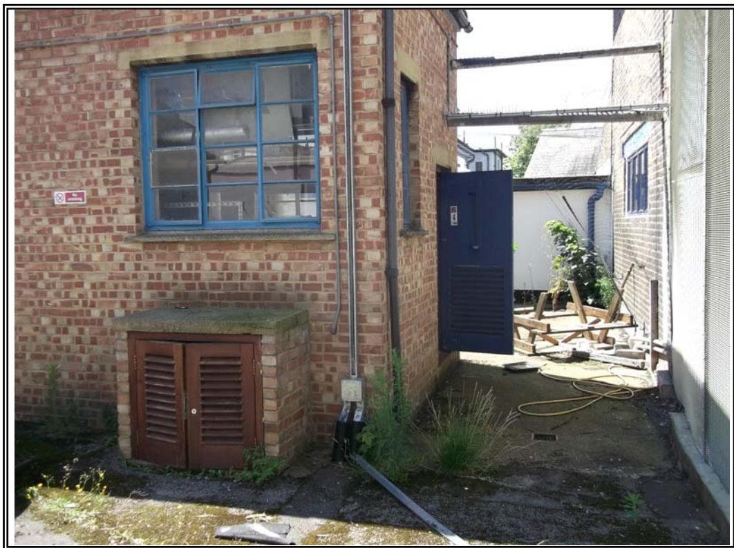
An old boiler house adjacent to the site entrance
