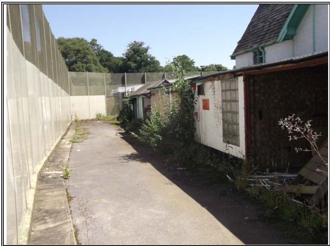
The rear of the works area
