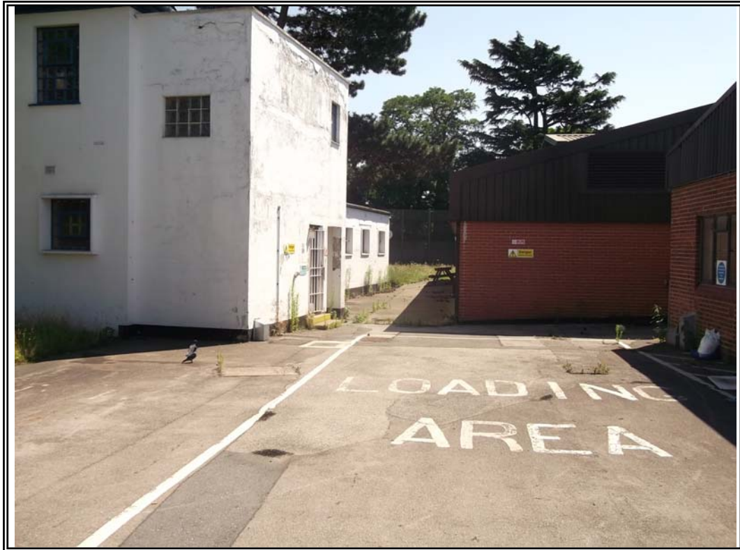
Northern end of the light assembly workshop
