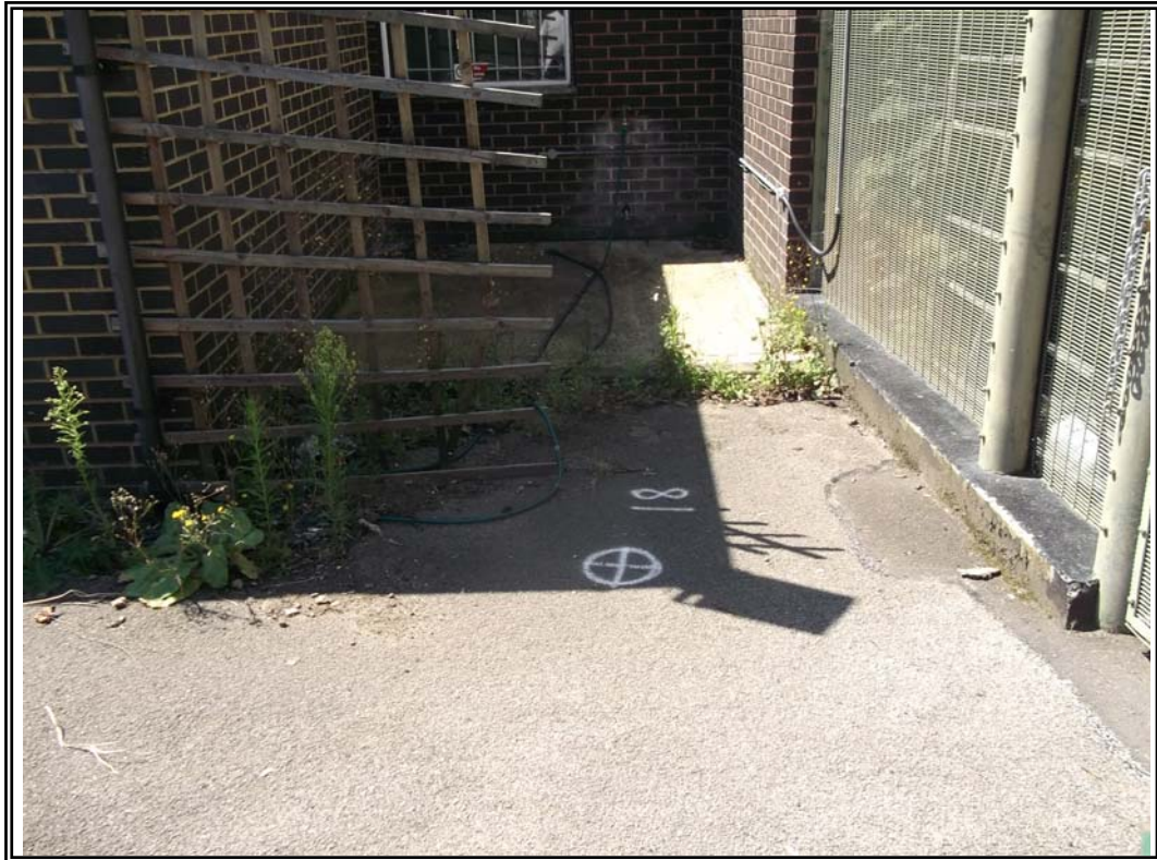
A potential above ground tank to the rear of the guard house
