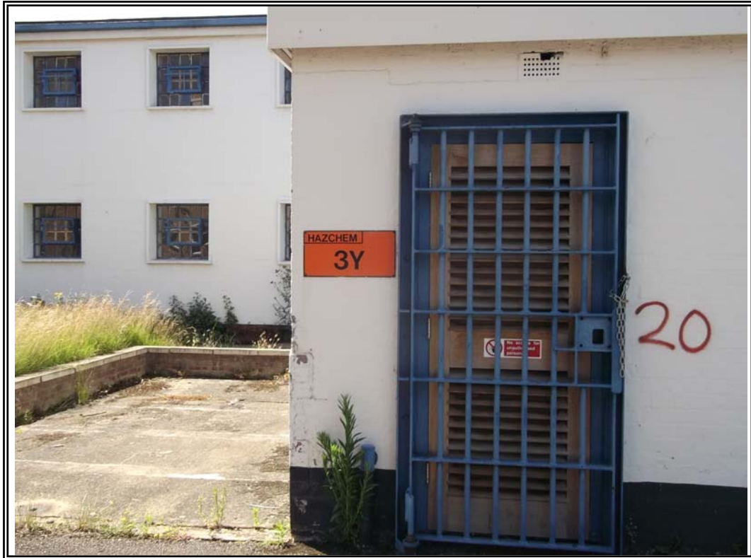
Hazardous chemical store and AST in main hard standing area.
