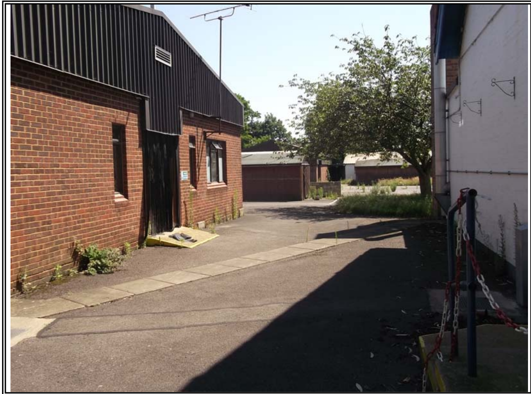
Light Assembly Workshop
