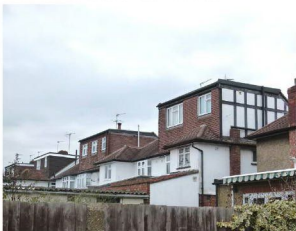
1 - 15 Garth Road rear extensions
