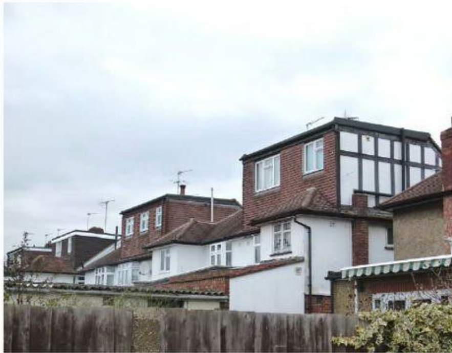
1 - 15 Garth Road rear extensions
