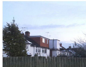
129 Latchmere Lane rear extension
