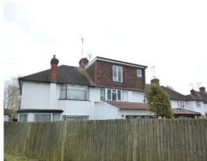
149 Latchmere Lane rear extension
