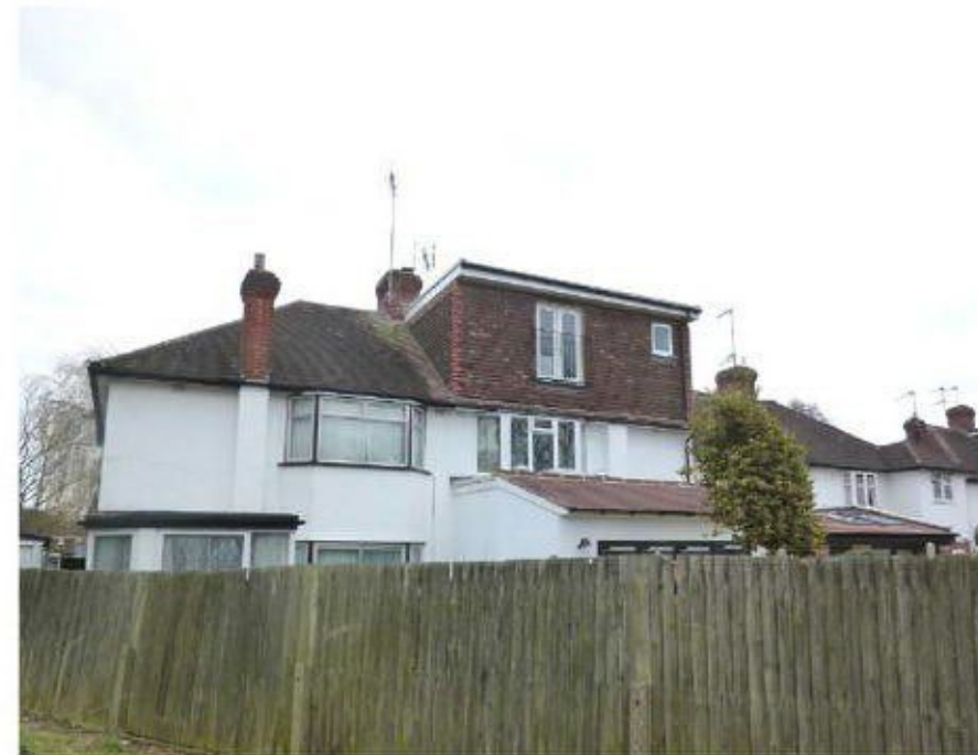
149 Latchmere Lane rear extension
