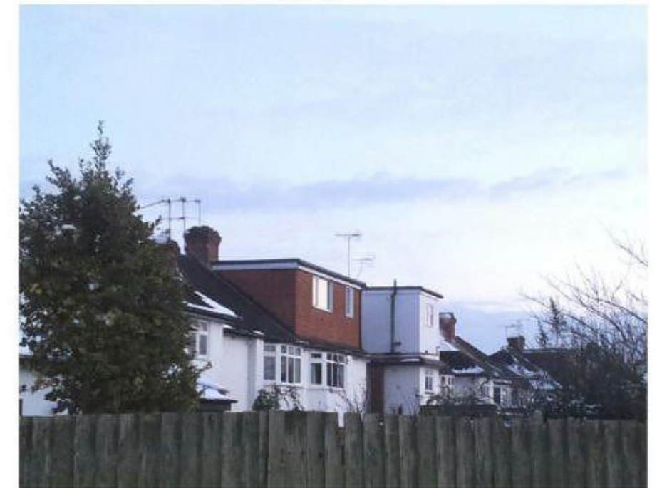
129 Latchmere Lane rear extension
