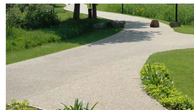
Gravel surface dressed paths
