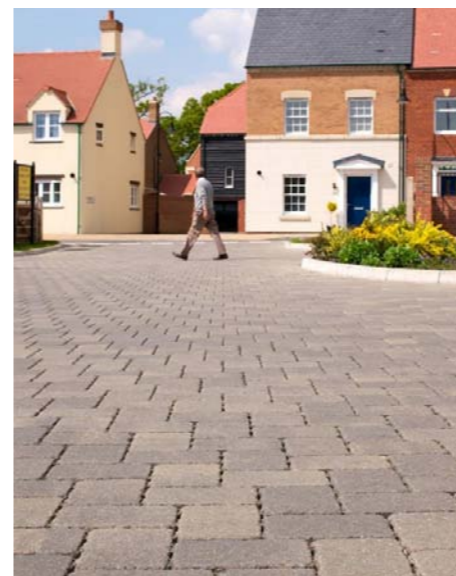
Permeable block paving
