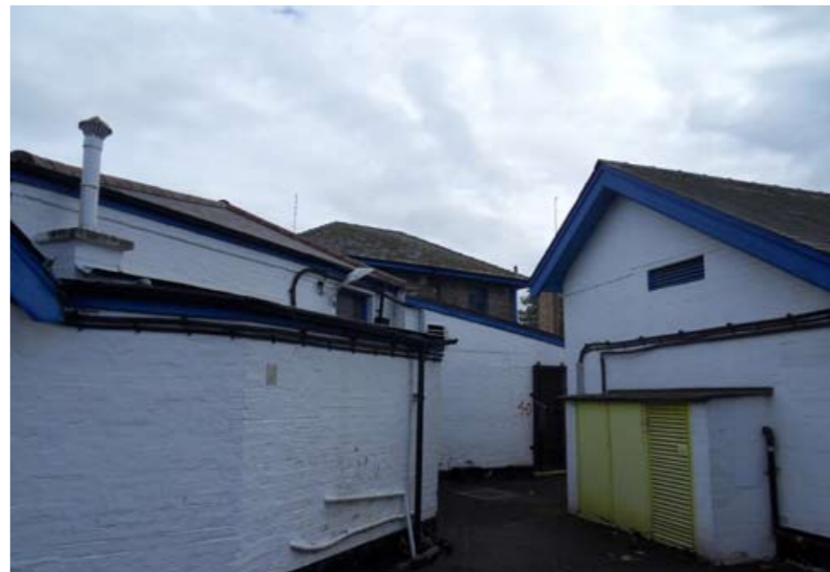
3. Eastern View from rear of additional buildings
