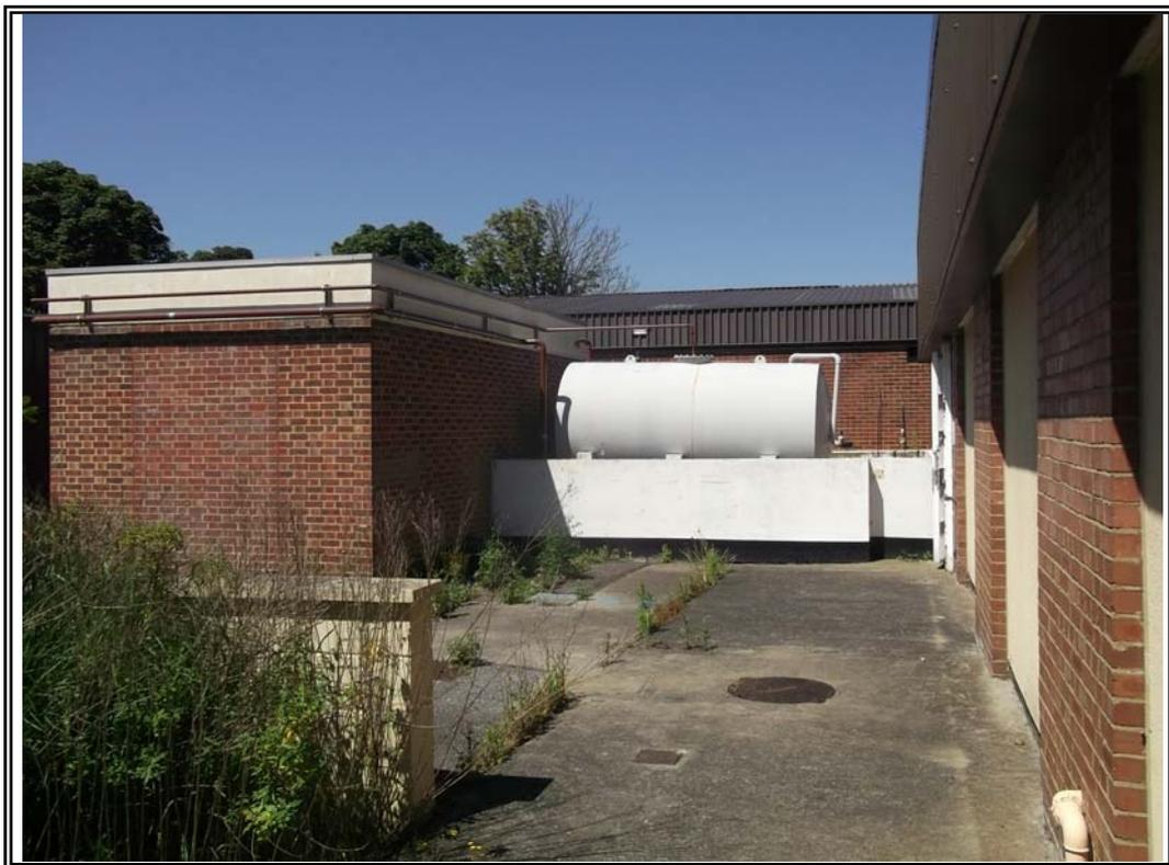
Above ground fuel tank for the emergency generator
