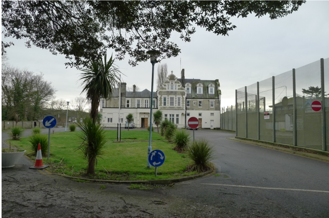
Figure 2: View of Latchmere House from north west within conservation area
