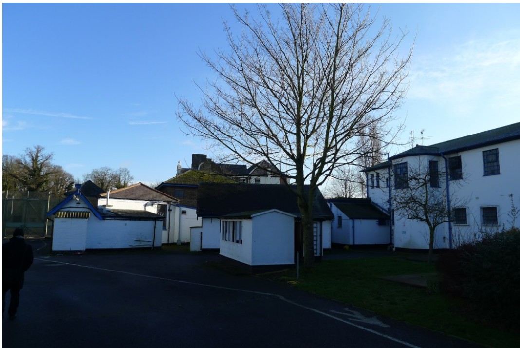
Figure 11: View towards Latchmere House from within remand centre site, including former 19 th /20 th century outbuildings and modern blocks in foreground
