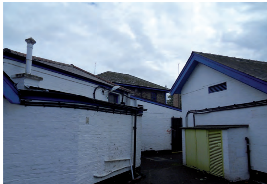
3. Eastern View from rear of additional buildings
