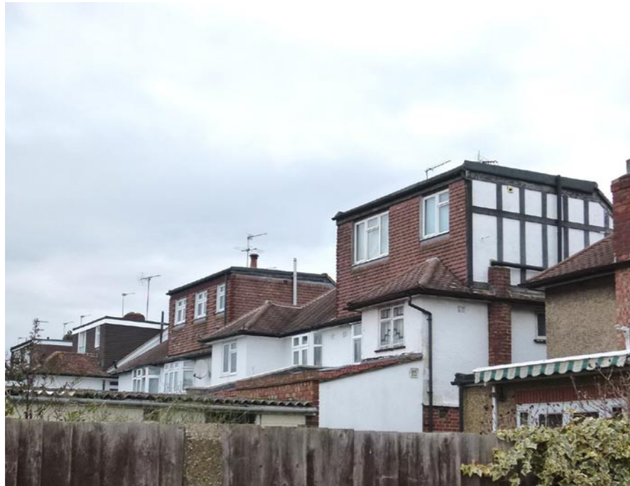
1 - 15 Garth Road rear extensions
