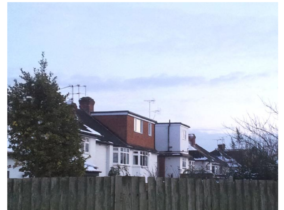
129 Latchmere Lane rear extension
