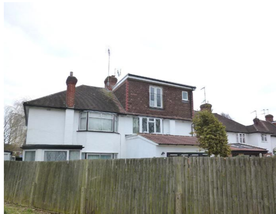
149 Latchmere Lane rear extension
