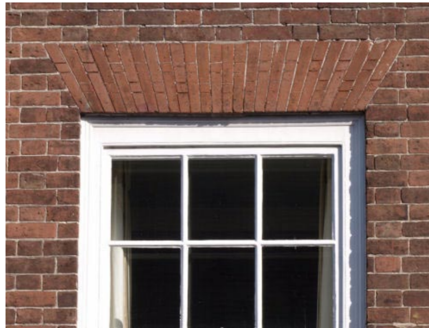
Window detail - Brick flat arch lintel
