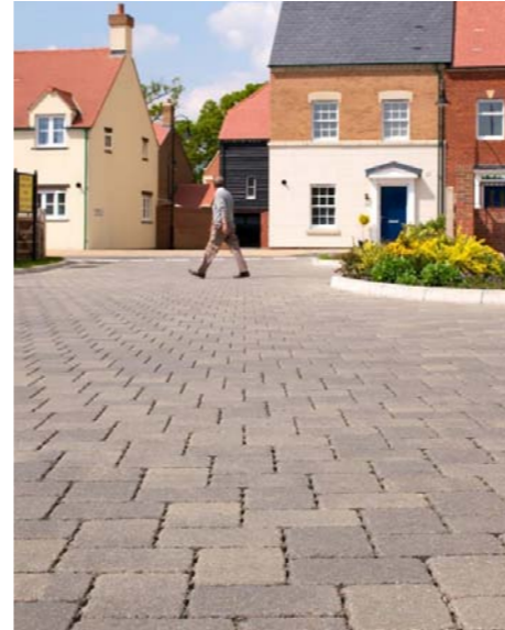
Permeable block paving
