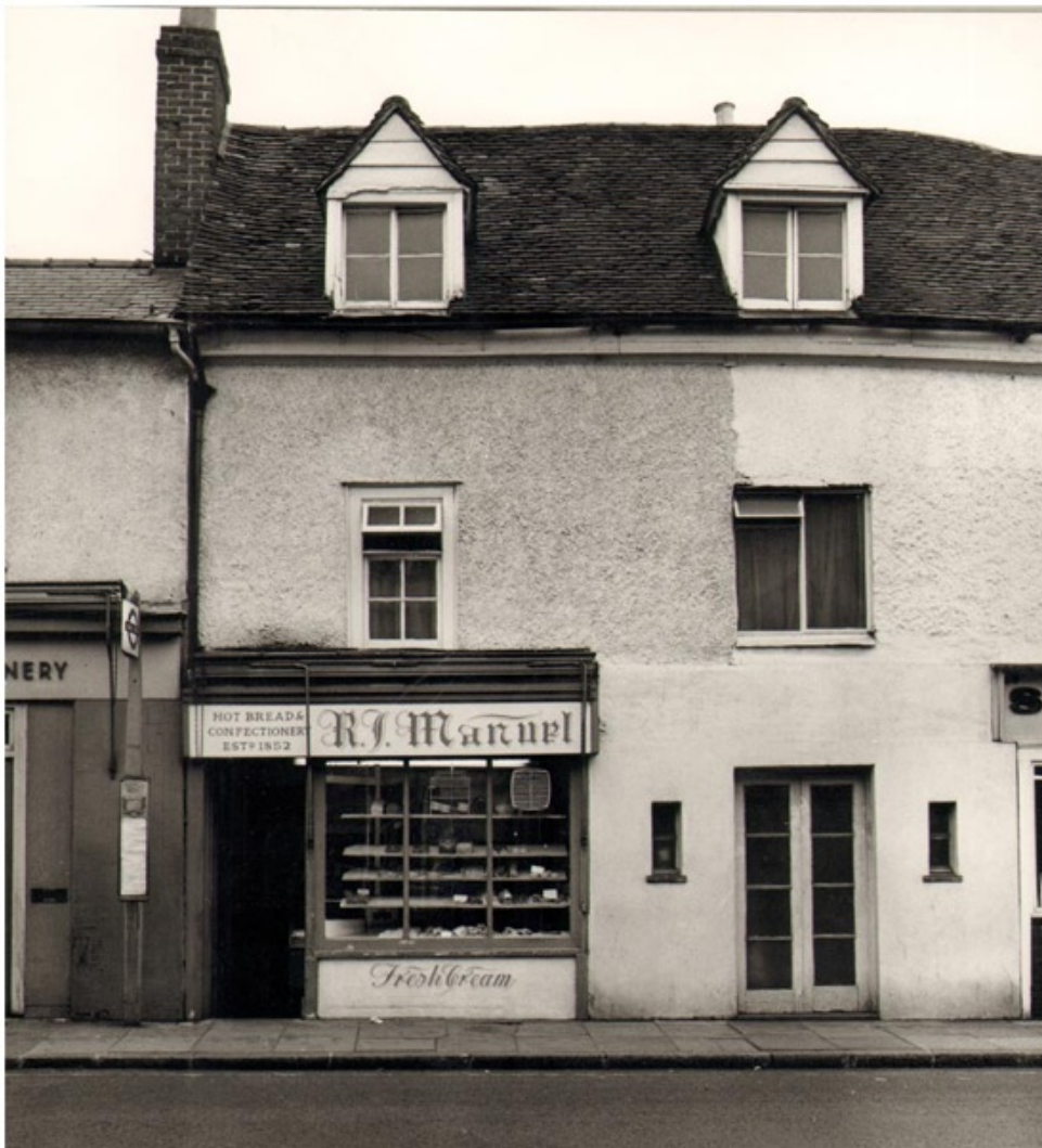
Plate 12 – 6-8 High Street before remodelling and boarding up
