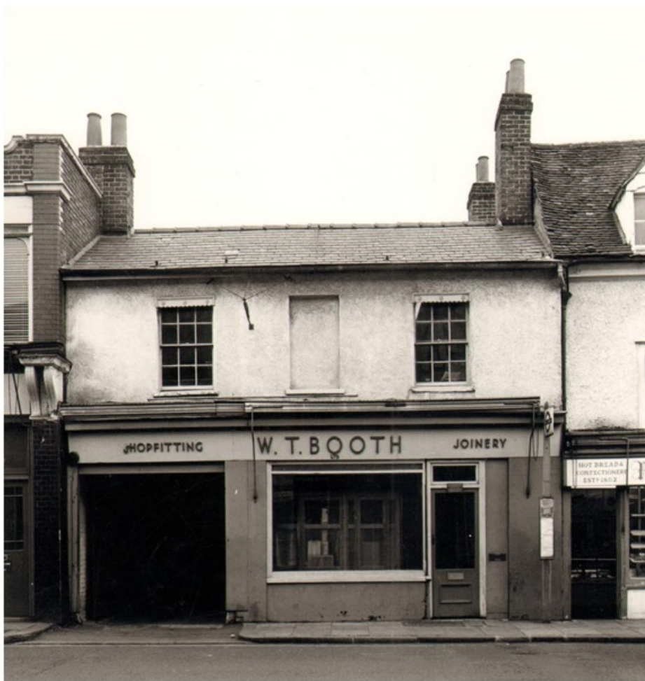
Plate 16 -10 High Street before remodelling and boarding up
