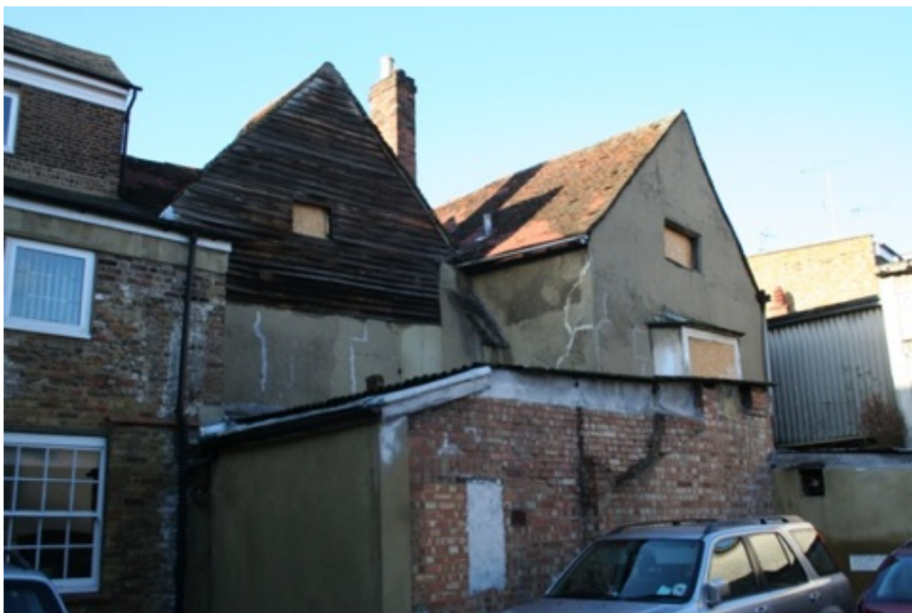
Plate 11 - East elevation of Numbers 6-8 showing seventeenth-century gables
