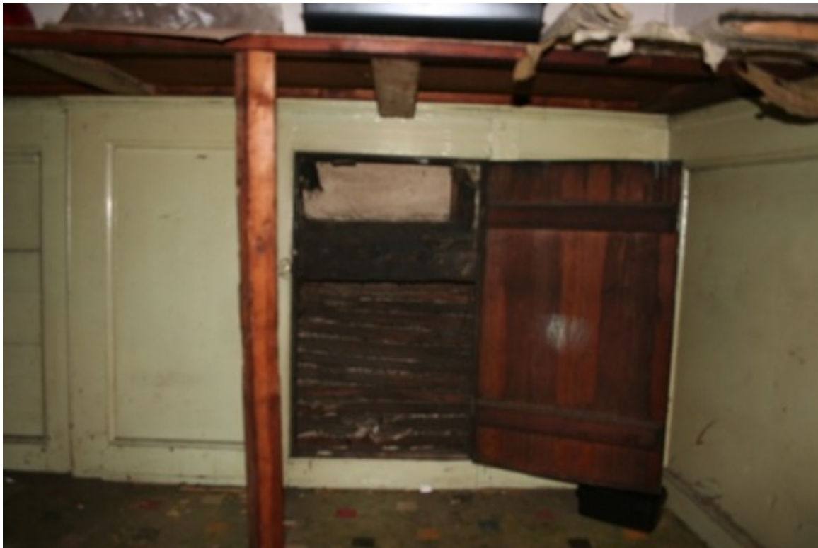
Plate 18 - Nineteenth-century panelling laid over original walling
