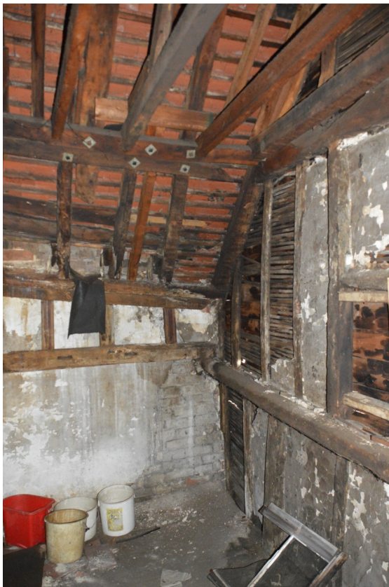
Plate 17 - Seventeenth-century roof and wall construction
