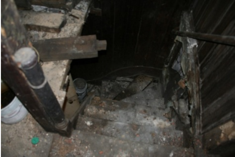
Plate 19 – Staircase with baluster newel post
