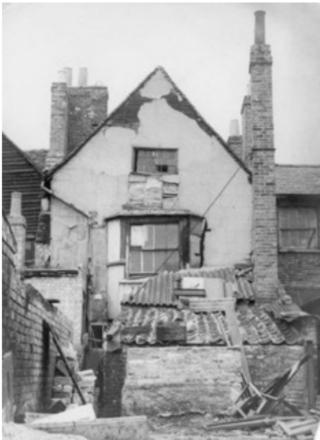
Plate 15 - Rear façade of Number 8 High Street in 1953
