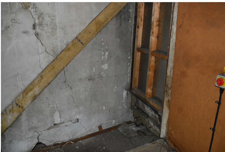
Plate 20 – Stairwell to attic floor
