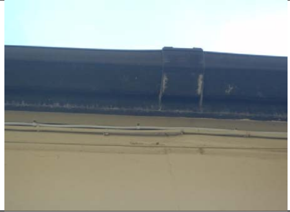
P20. The sealed soffits of Building 5.
