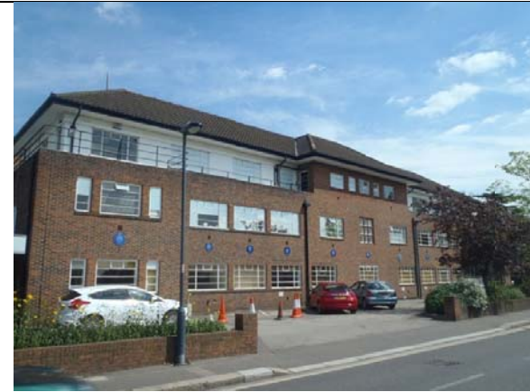
P7. Building 3 viewed from Broom Road to the south west.
