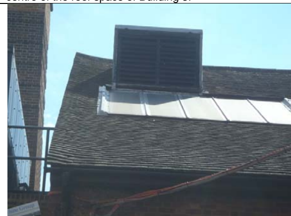
P15. The tiled roof of Building 4 viewed from the north west showing slightly raised tiles on the verge.
