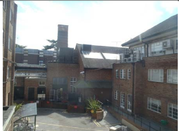
P14. Building 4 viewed from the north west.
