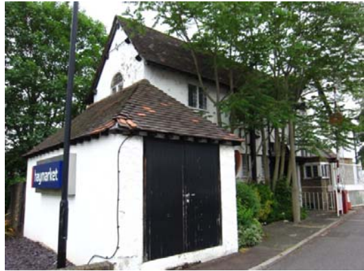
P2: Building 1 – cottage in south western corner of site
