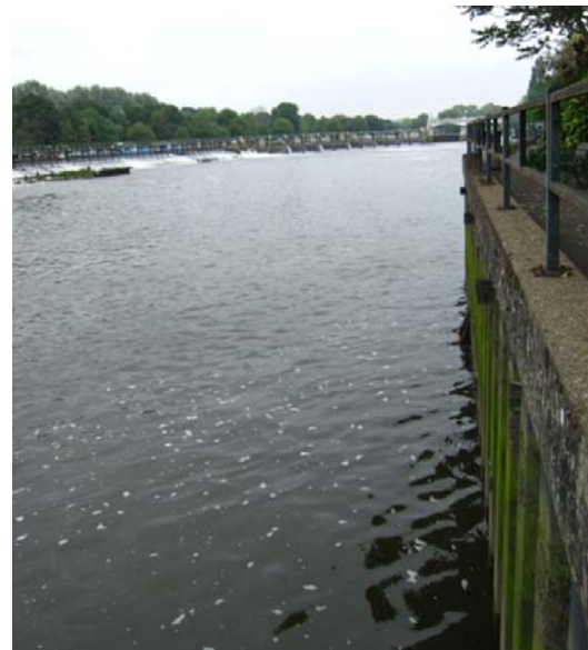
P6: Sheet pilings at northern boundary of site with River Thames
