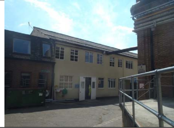
P19. Building 5 viewed from the north showing the corrugated sheet roof and rendered walls.
