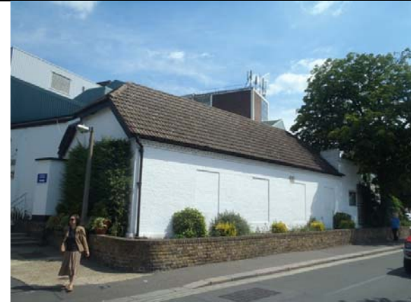
P1. Building 2 viewed from Broom Road to the south west.
