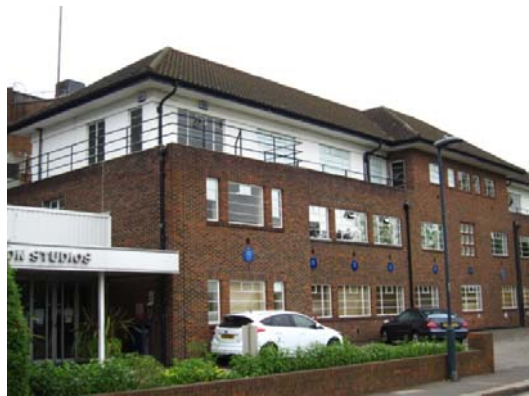
P4: Building 3 and ornamental shrubs at southern boundary of site
