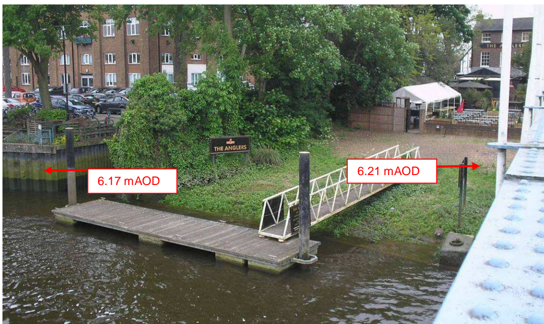
Figure B-13 Existing defences on Teddington bank above 6.1 mAO (5% level at 6.06 mAO)
