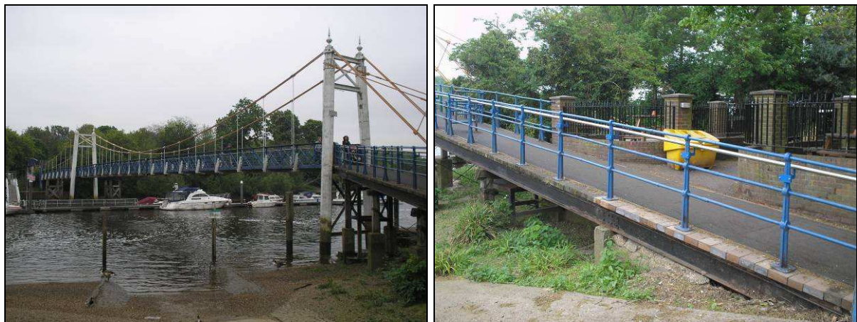
Figure B-10 Teddington Lock Footbridge showing existing access from the Anglers' Arms
