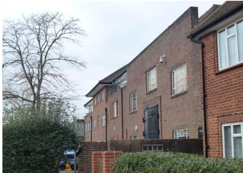
Figure 6: The main Administrative Block (to the rear), and Boiler House of Teddington Studios, originally built as part of Warner Brothers' investment into the site from 1934 onwards.
