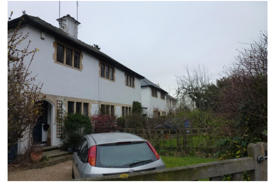
Figure 49: 1-9 Kingston Road, viewed from the corner with Ferry Road.
