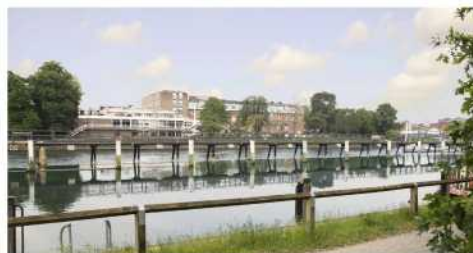
Visual showing existing site across Teddington Weir
