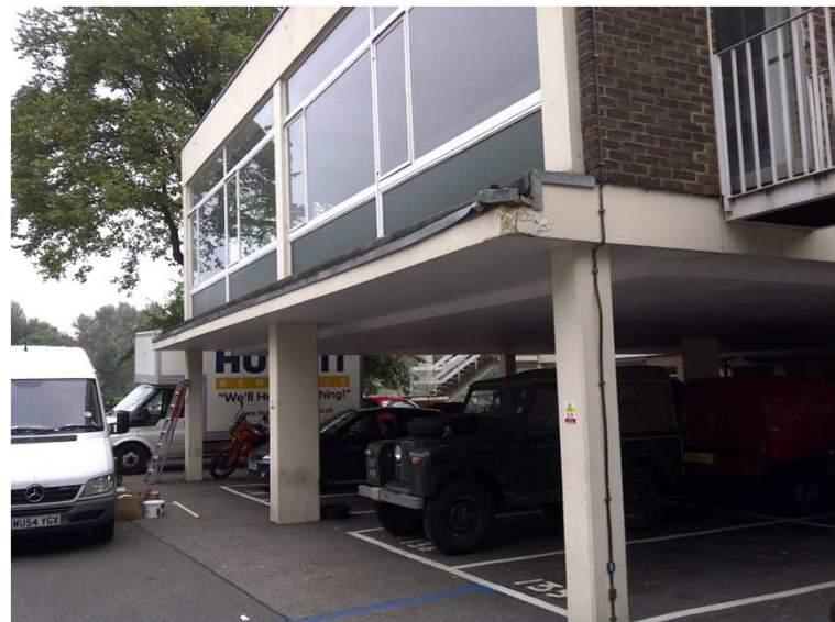
Image 16: Building on the north-east of the site with undercroft parking
