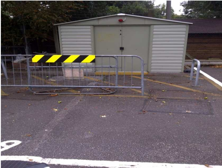
Image 9: Below ground sewage tank on the east of the site
