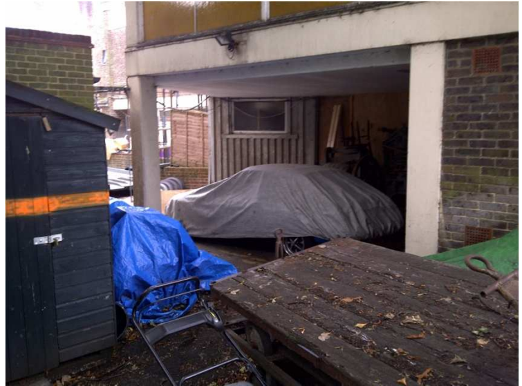
Image 10: Building to the north-east with undercroft parking
