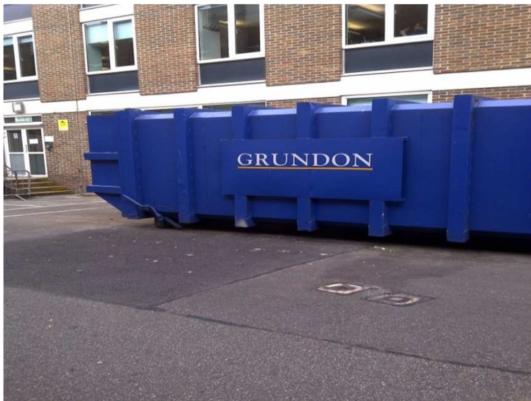
Image 15: Skip with general construction waste in front of north-east building
