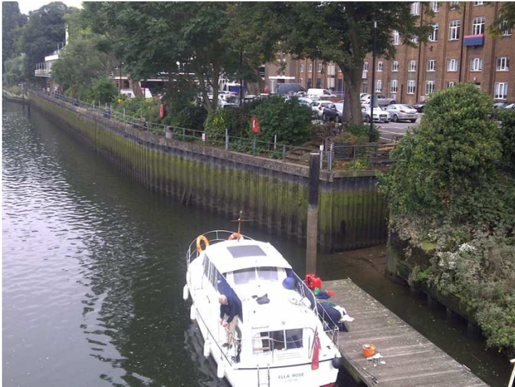
Image 3: Retaining wall view from the bridge
