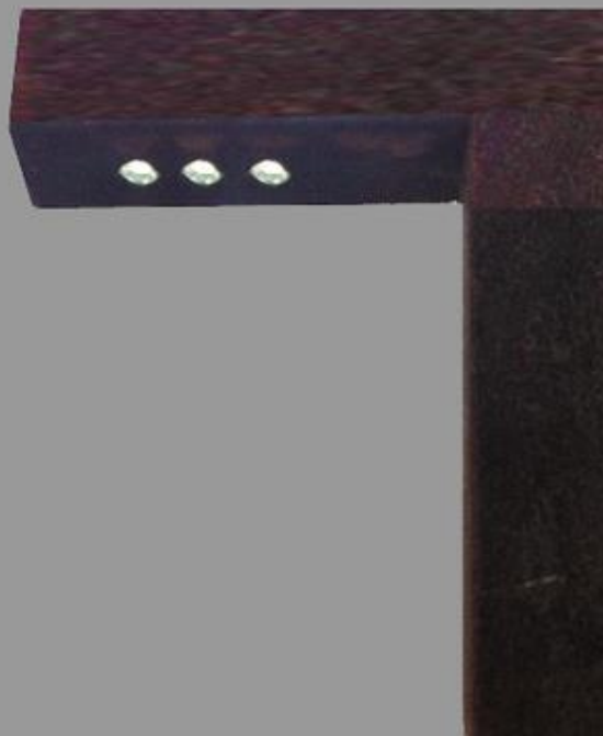
Dark Sky Compliant External Lighting
