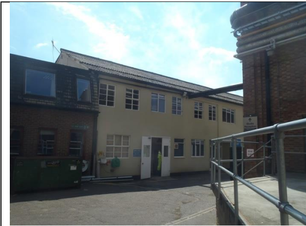
P19. Building 5 viewed from the north showing the corrugated sheet roof and rendered walls.
