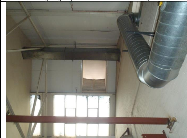
P17. The boarded roof, skylights and vent in the boiler room of Building 4.
