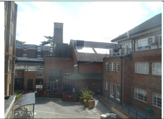
P14. Building 4 viewed from the north west.
