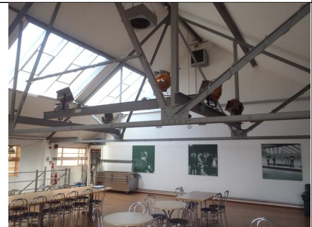
P18. The open roof and skylights within the café in Building 4.
