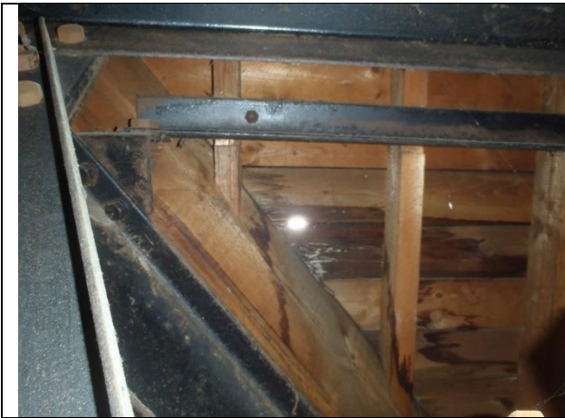
P13. Daylight visible between the sarking boards in the centre of the roof space of Building 3.
