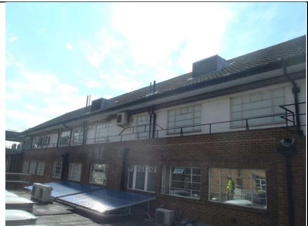
P8. Building 3 viewed from the flat roof to the north east.
