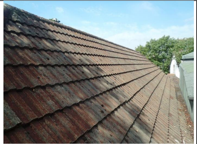
P2. The tightly fitting concrete roof tiles on Building 2.
