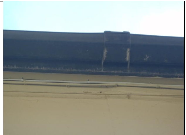
P20. The sealed soffits of Building 5.
