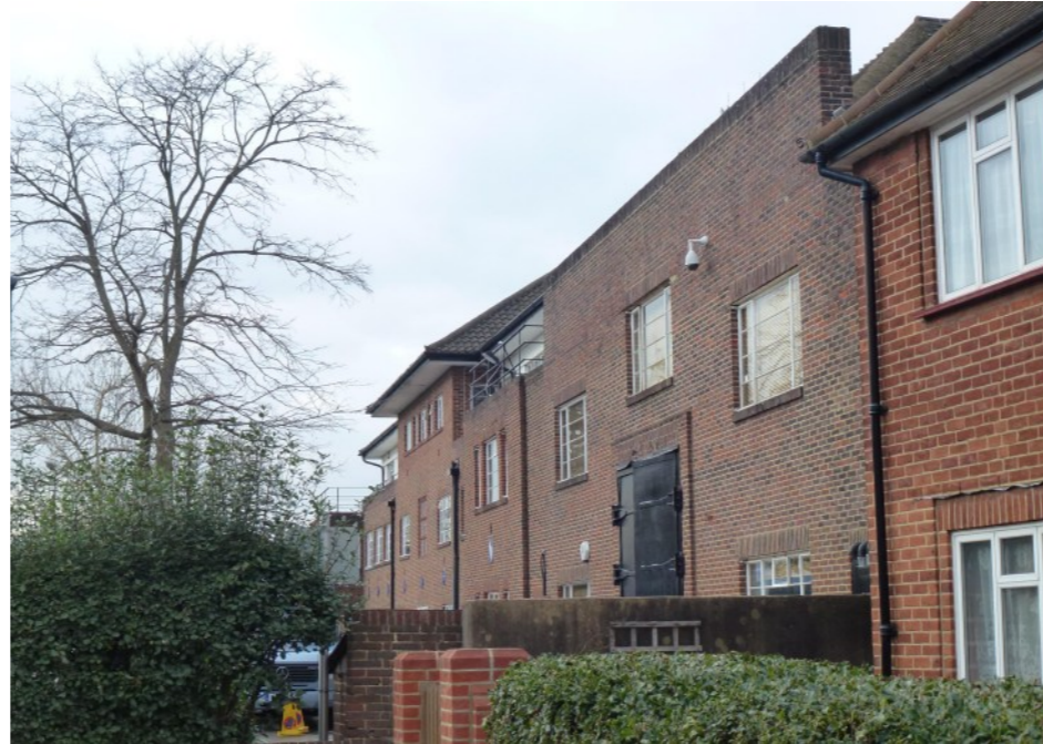
Figure 6: The main Administrative Block (to the rear), and Boiler House of Teddington Studios, originally built as part of Warner Brothers' investment into the site from 1934 onwards.
