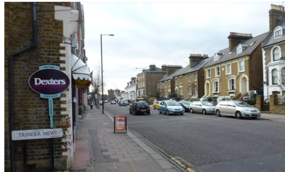
Figure 3: Teddington High Street, showing its largely Victorian fabric, illustrating the boom was felt during the nineteenth century, as it changed from a village of 800, to a town of nearly 7,000 within 100 years.
