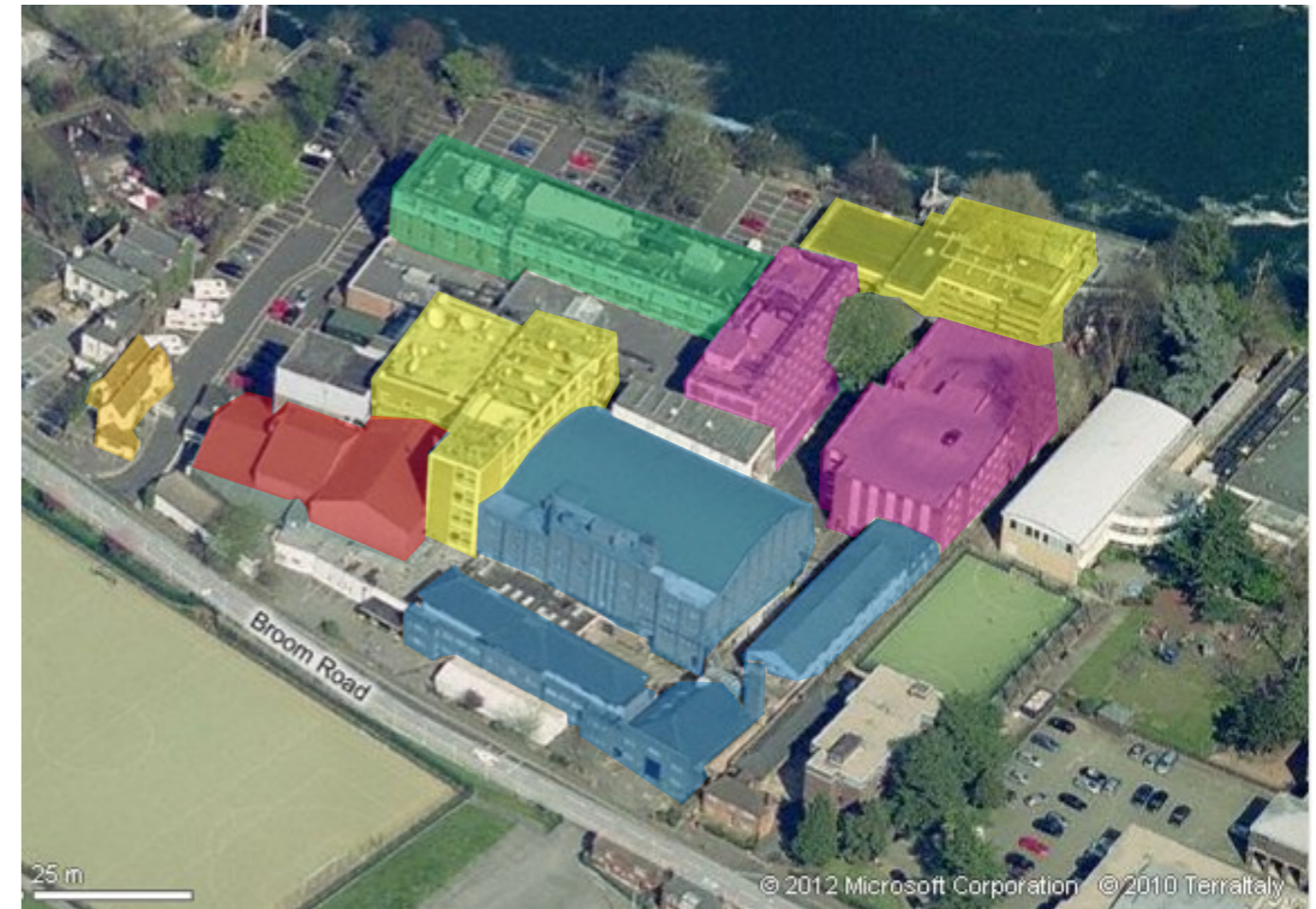
Figure 25: Aerial image of Teddington Studios, with the ages of the main buildings on the site indicated, according to the colour coding described to the left. It should be noted that while Studio 1 dates in design to the 1930s, it was actually almost entirely rebuilt, according to its original design, between 1946 and 1948.
