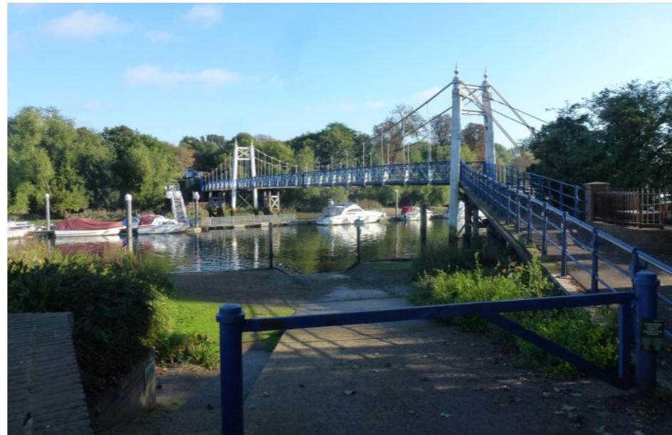
Figure 33: Teddington Footbridge, viewed from the bank. Only the Teddington side of the structure can be seen here.
