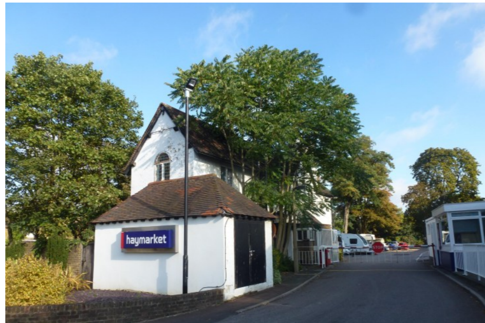
Figure 43: Weir Cottage, viewed from Broom Road.
