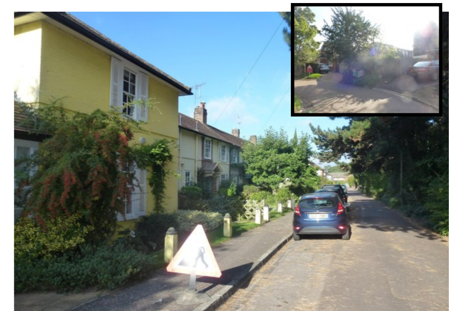
Figure 32: Typical view of the Grove Conservation Area, with (inset), the view towards the development site, showing the extent to which it is screened visually.
