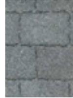
Permeable block paving to piazza with conservation kerb - eg graphite Mistral by Marshalls
