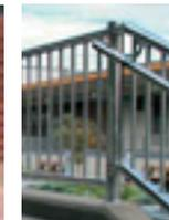
1100mm high railing to riverside walk and ruefurbished flood wall
