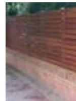
1100mm high brick wall to compliment building with quality timber panel fence on top
