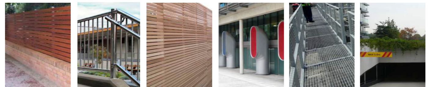
1100mm high brick wall to compliment building with quality timber panel fence on top 1100mm high railing to riverside walk and refurbished flood wall Slatted timber panel fence Car park ventilation Safe access/egress walkway Vegetated entrance to undercroft car park
